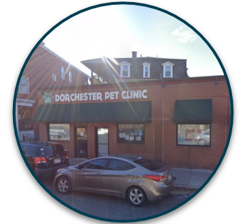
Some small offices on the ground floor
