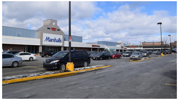
Image of parking lot and retail uses located within the Border Street DPA
