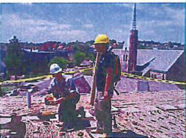
Saint Polycarp Village (Green Roof Installation)
