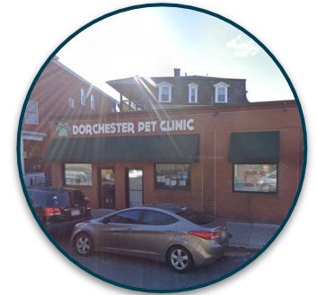
Some small offices on the ground floor
