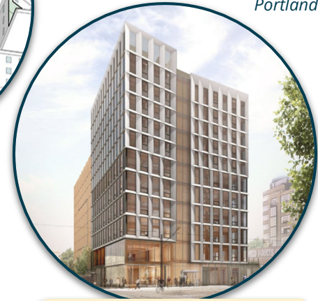
Mixed-use mass timber 12-story building in Portland
