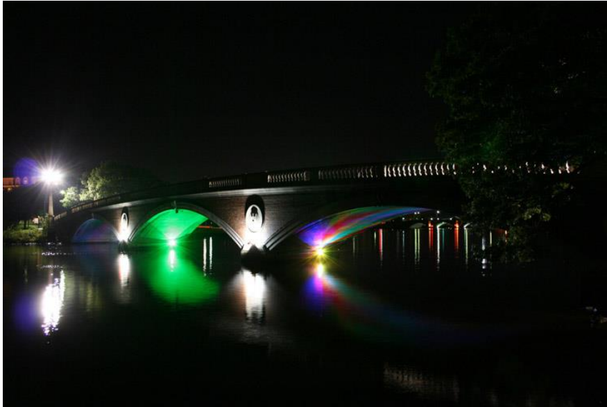
Weeks Footbridge crossing the Charles River. Working with Luminous Technologies in Woburn, MA and the Charles River Conservancy in 2008 the first bridge crossing the Charles River to be lit with purpose built LED fixtures
