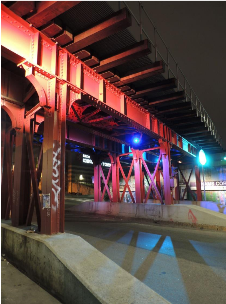
Uphams Corner bridge lighting, at the Uphams Corner T stop, commissioned by the Boston Foundation through the Dudley Square neighborhood Initiative and the Design Studio for Social Intervention
