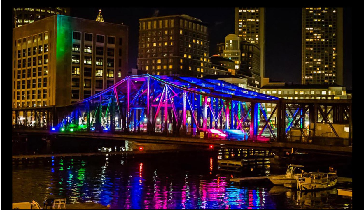
OLD NORTHERN AVENUE BRIDGE, BOSTON, 2014 CITY OF BOSTON, DEPT OF PUBLIC WORKS AND LIGHTBOSTON DESIGNER: JOHN POWELL
