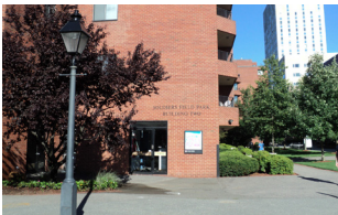
Existing Building 2 Entrance
