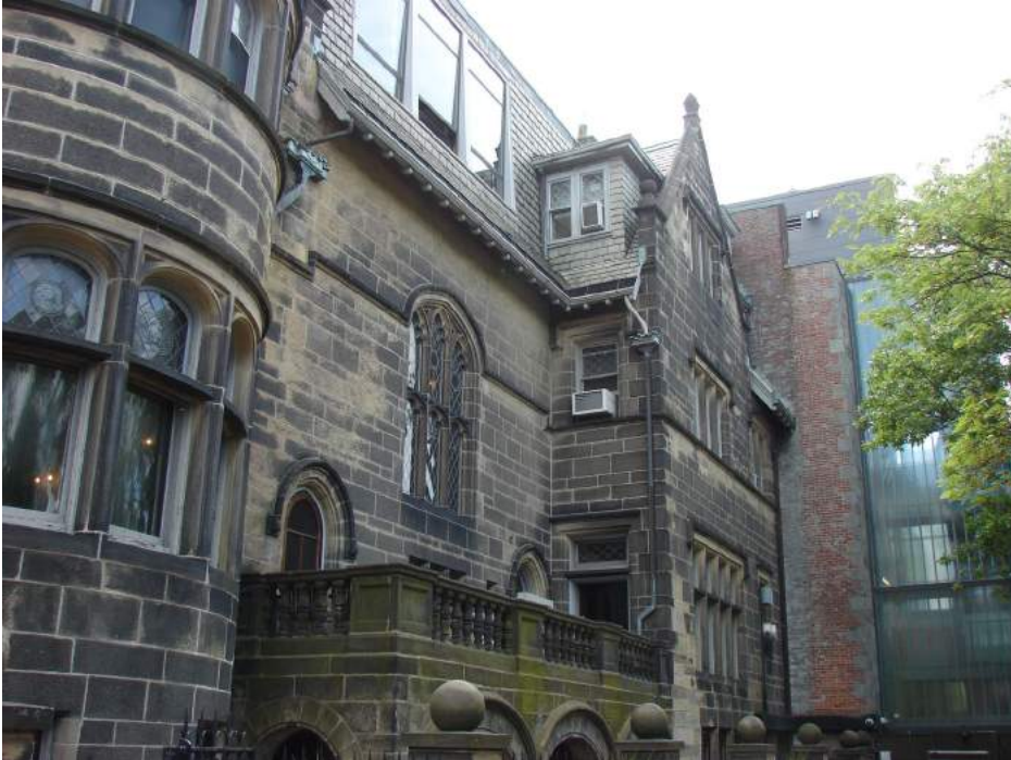
Photograph 3: View of rear facade looking southwest
