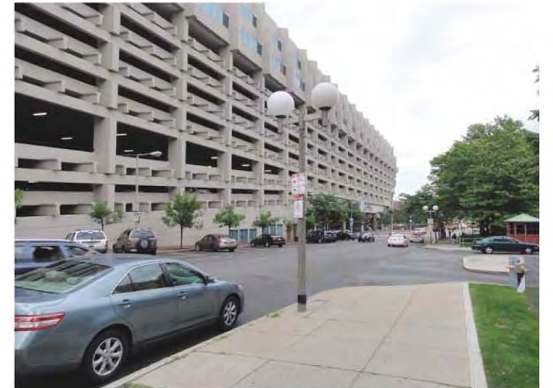
View from New Sudbury Street
