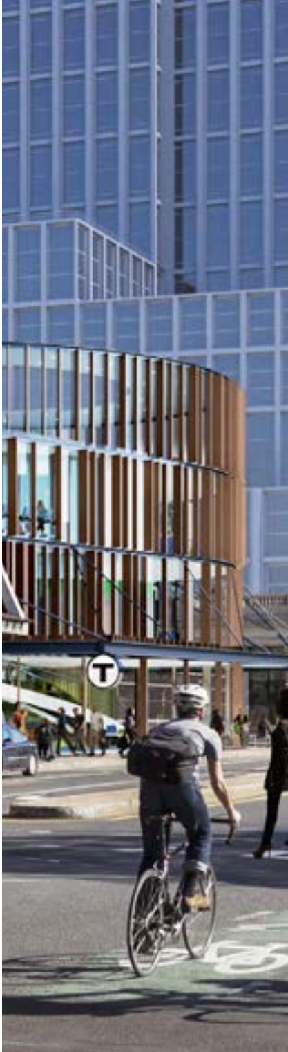
View of enhanced MBTA station at Massachusetts Avenue
