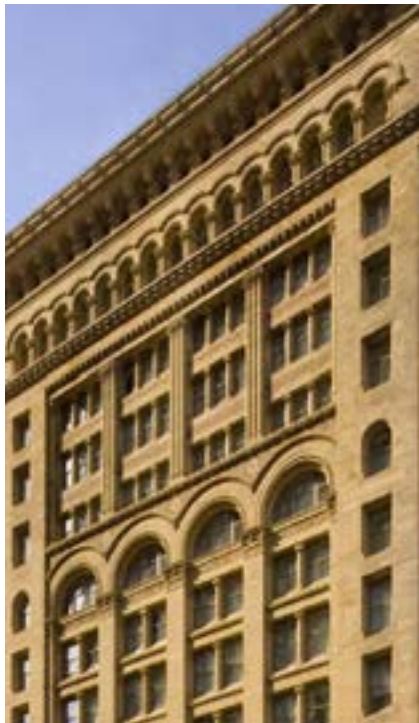
Ames Building renovation by Tishman Designed by C7A
