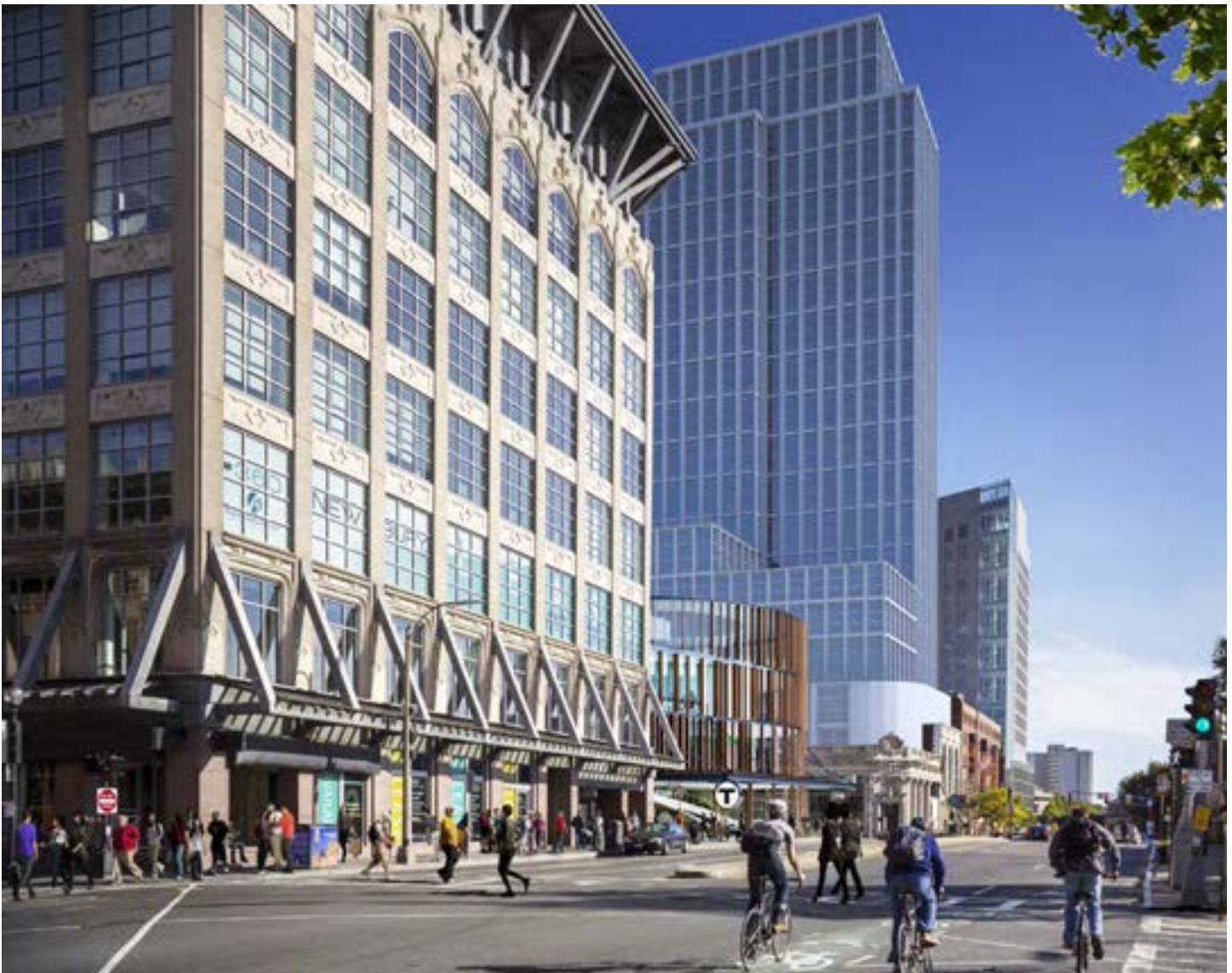
View 2: Massachusetts Avenue looking south
