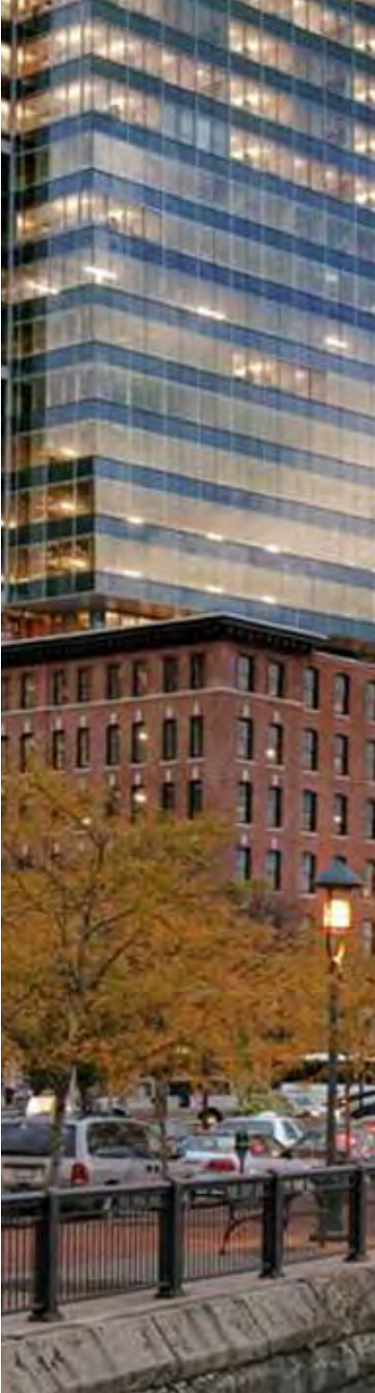
Atlantic Wharf Structural engineering by McNamara/Salvia
