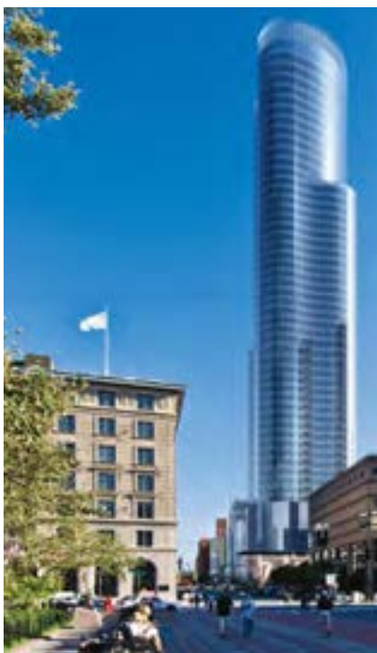
Copley Tower developed by BRG Structural engineering by McNamara/Salvia
