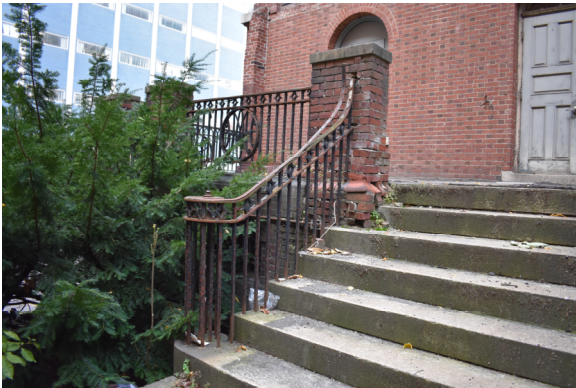
1. Cast iron railing is in poor condition and the brick pier has significant mortar loss and rust jacking.
