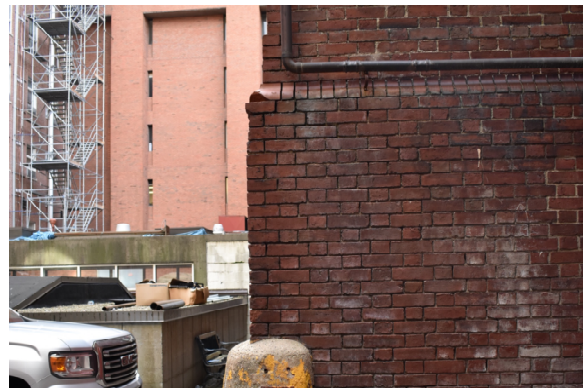
4. Several bricks at the north corner are chipped or have spalls. Area also has numerous open and deteriorated mortar joints.
