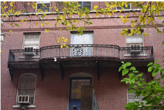
3. Original cast iron balcony with some deterioration.
