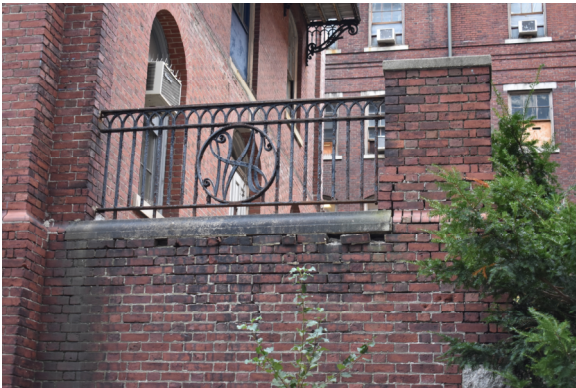
1. Area of missing and displaced brick under cast iron railing. Area also shows deteriorated and open joints.
