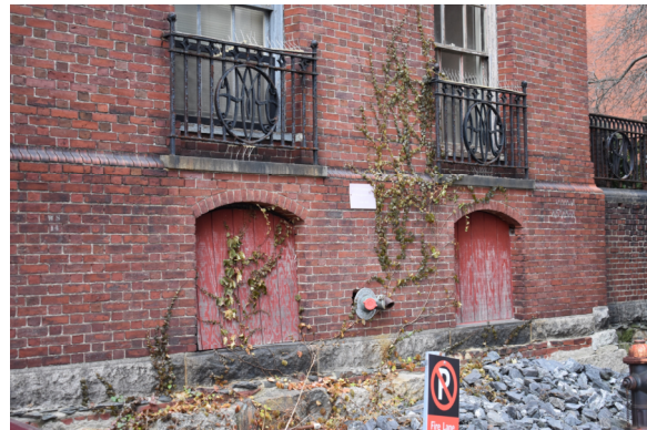
2. Deteriorating paint and wood board over basement windows, along with soiling on limestone and granite and vegetation growing on brick wall.
