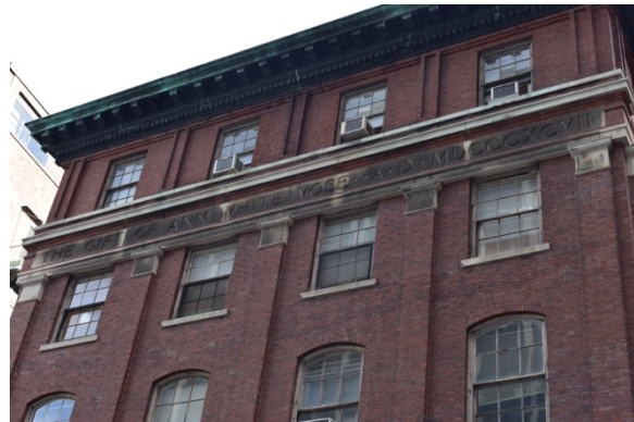
2. Limestone inscription band is in good condition despite heavy soiling. Copper cornice above is missing components and has open seams.
