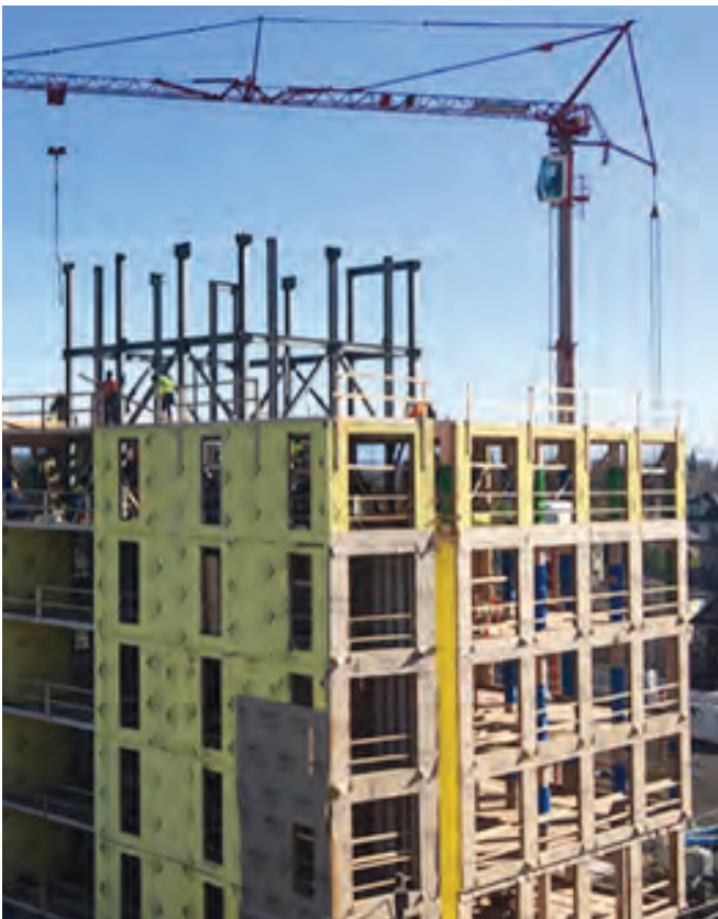
Completed in 2018, Carbon12 was engineered using an innovative steel brace frame core surrounded by a timber and CLT structure
