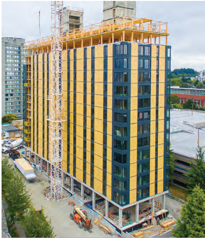
Brock Commons Tallwood House Vancouver, Canada | 17 stories of mass timber over a concrete podium, with two concrete stair cores Architect: Acton Ostry Architects Structural Engineer: Fast + Epp Structural Engineers
