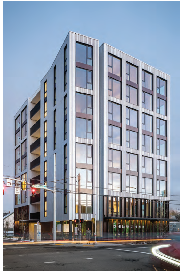
Carbon12 Portland, Oregon | Eight stories of mass timber Kaiser Group and Path Architecture Munzing Structural Engineering
