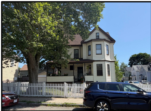
Existing homes with no driveway would be illegal to build today.
