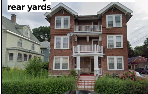
Driveways in side yards are common
