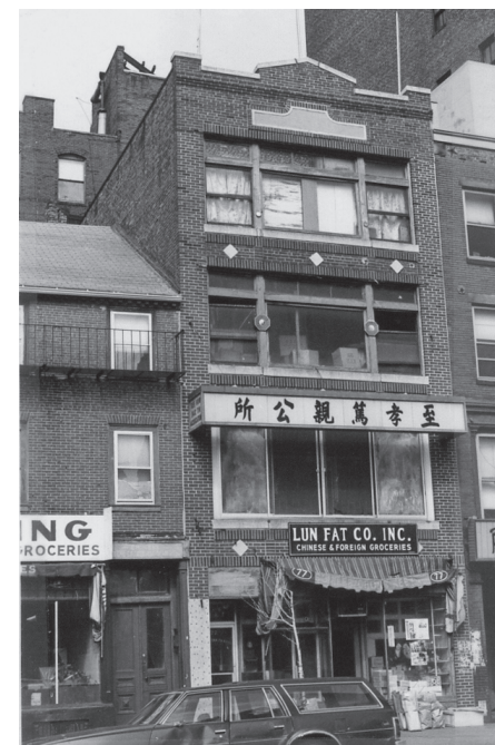
77 Harrison Avenue, 1979 (source: MACRIS)
