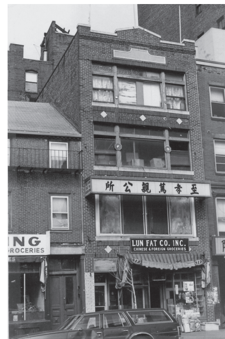
77 Harrison Avenue, 1979 (source: MACRIS)
