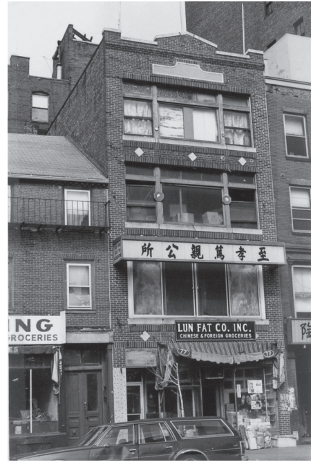
77 Harrison Avenue, 1979 (source: MACRIS)
