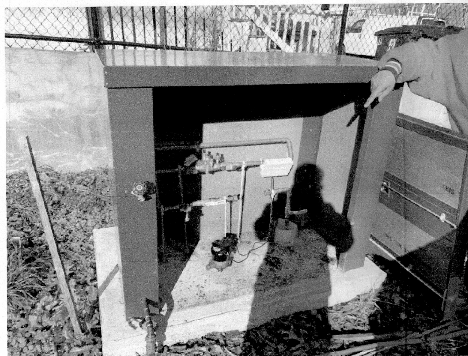
TYPICAL HOT BOX (HB) DETAIL
