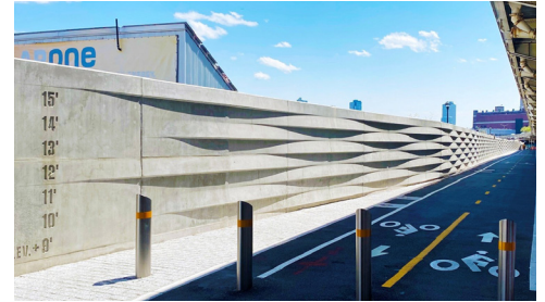
Flood wall with architectural concrete finish in the East Side Coastal Resiliency project in NYC (Source: OFTN Architecture)
