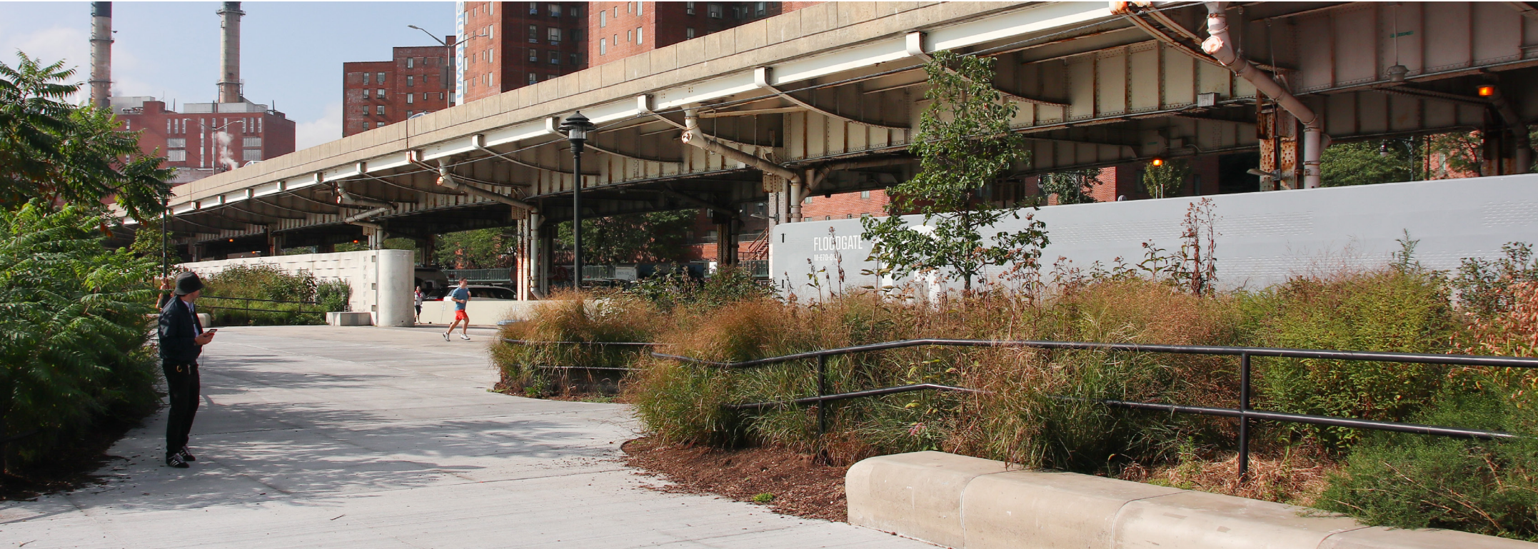
Movable flood gate in the East Side Coastal Resiliency project in NYC. Active floodproofing requires human intervention to provide flood protection (Source: OFTN Architecture)
