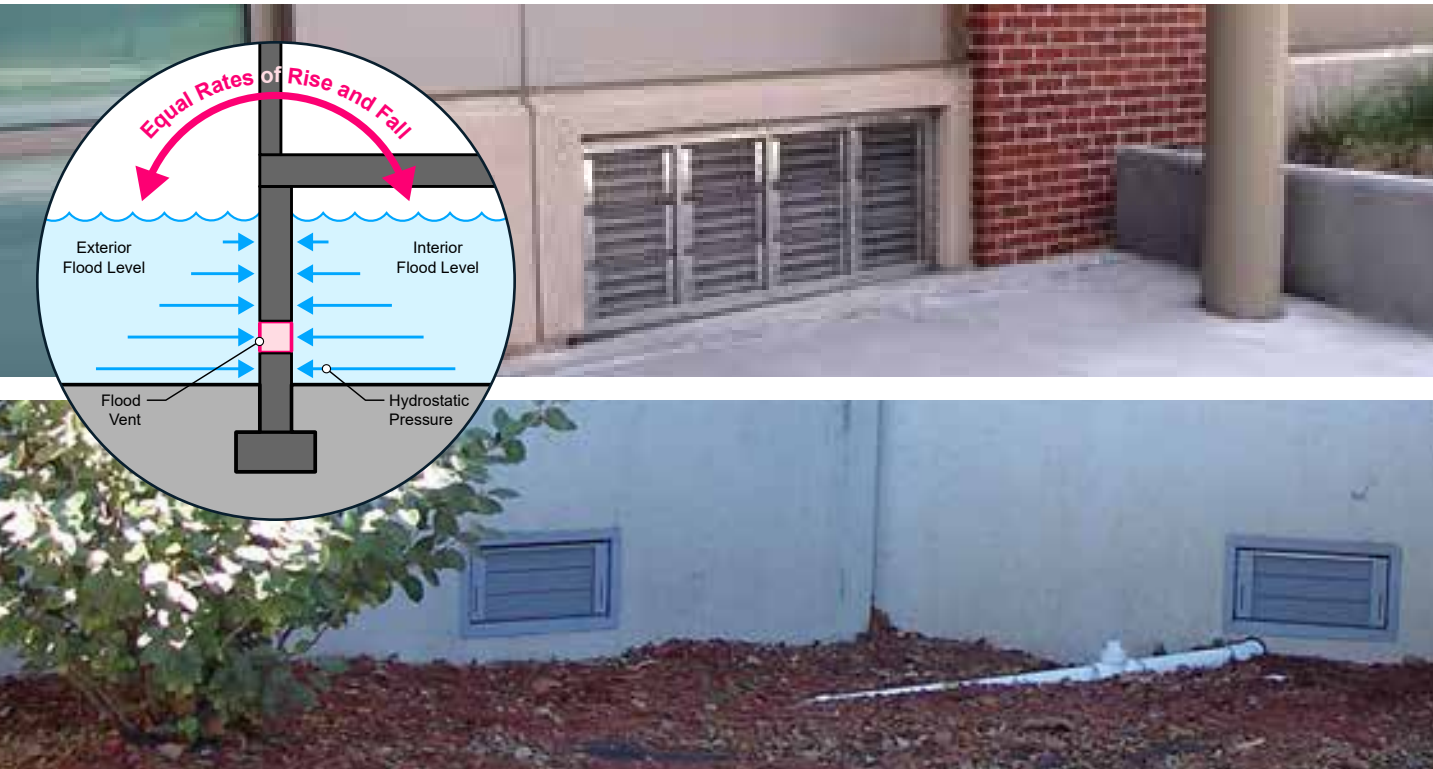
Wet floodproofing designs for the movement of water through an uninhabited space or a building, which equalizes hydrostatic pressure and helps prevent structural failure. Involves use of flood vents or other openings and flood-damage-resistant materials. (Source: Continuing Education Centers/ Photo by Smart Vents, Inc. (top), FEMA (bottom))
