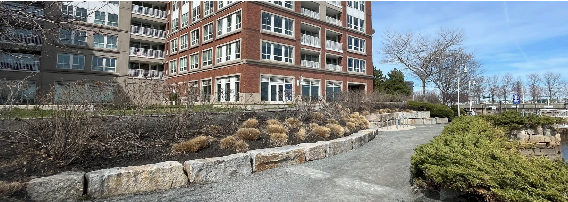
Upper level harborwalk (left) acting as flood barrier at Charlestown Harborview. Passive floodproofing is permanently installed and provides 24/7 asset protection without any electricity, personnel, or training (Source: OFTN Architecture)
