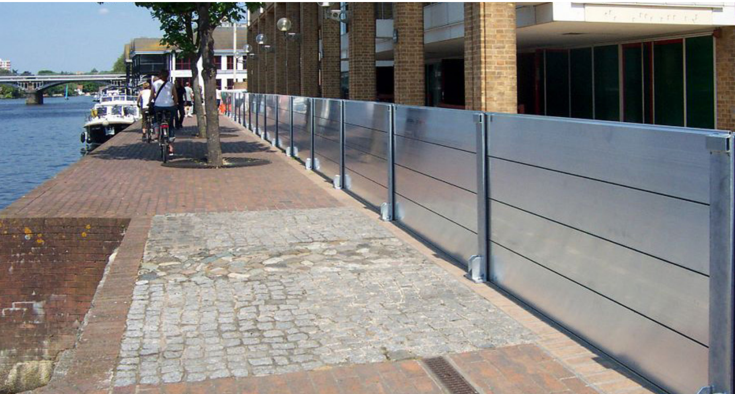
Dry floodproofing seals a space or a building to eliminate or reduce potential flood damage by keeping floodwaters out of the structure. Involves use of active or passive flood barriers at openings or around the perimeter of a building. (Source: Flood Control International)
