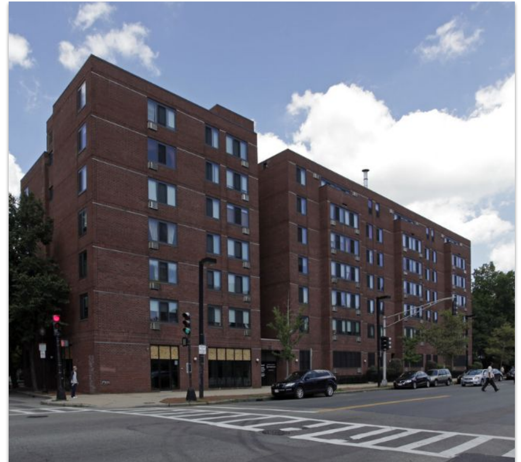
RC-4 + RC-5: The Concord Houses, South End
