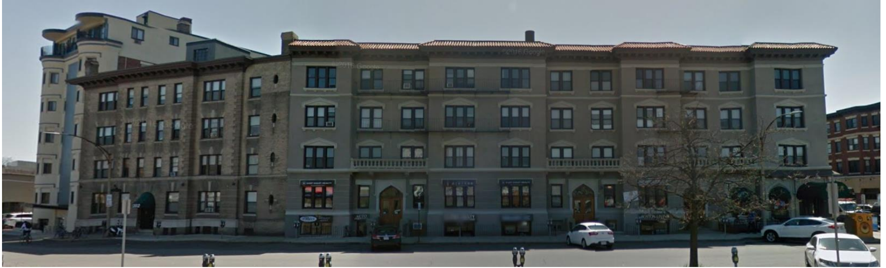
Directly west of the site - 1200 Commonwealth Avenue to Harvard Avenue
