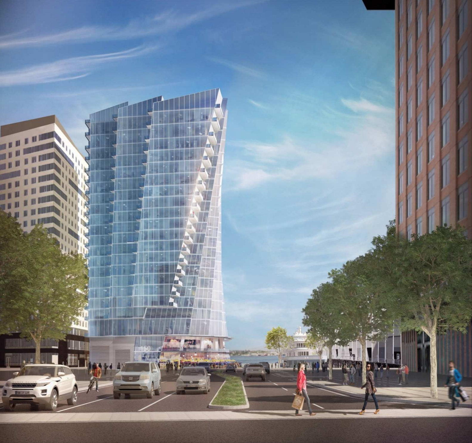
View from B Street
