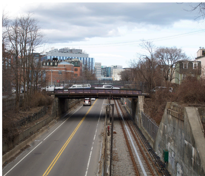
FIG 166 : EXISTING HAUL ROAD BRIDGE AND DORMANT FOOTING
