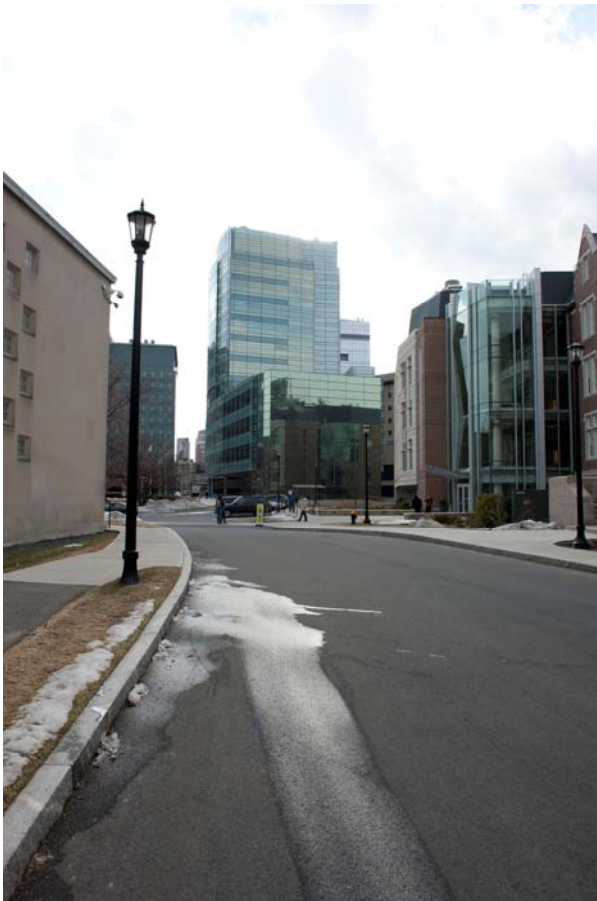
The Merck Research Laboratories-Boston and Wilkens Science Center buildings provide visual focal points from the east Institutional Gateway on The Fenway.
