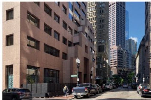
Large-scale commercial buildings in the Financial District
