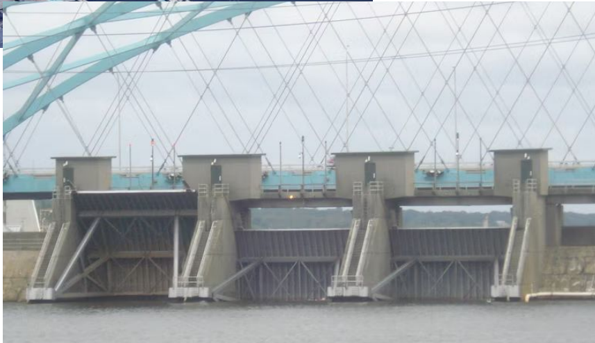
Fox Point Hurricane Barrier, Providence, RI Image source: USACE, New England District
