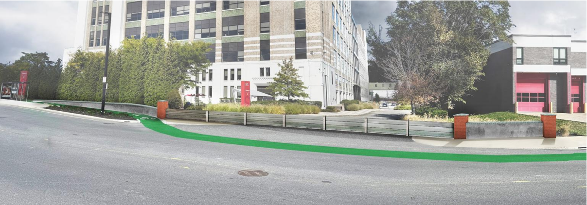
Expected appearance of kneewall with deployable stop logs (Charlestown - Main St.)
