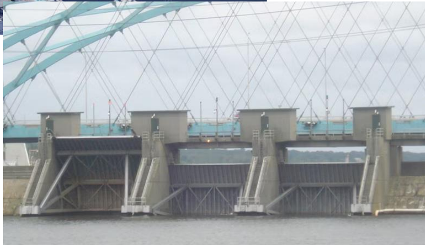
Fox Point Hurricane Barrier, Providence, RI Image source: USACE, New England District
