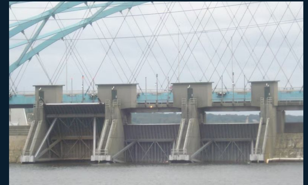
Fox Point Hurricane Barrier, Providence, RI Image source: USACE, New England District
