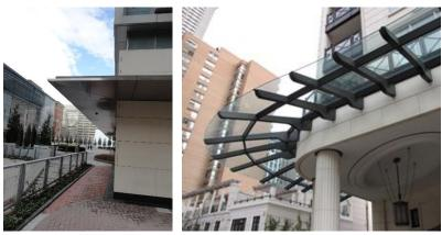
Image 2 - Examples of canopies wrapping around the building corner
