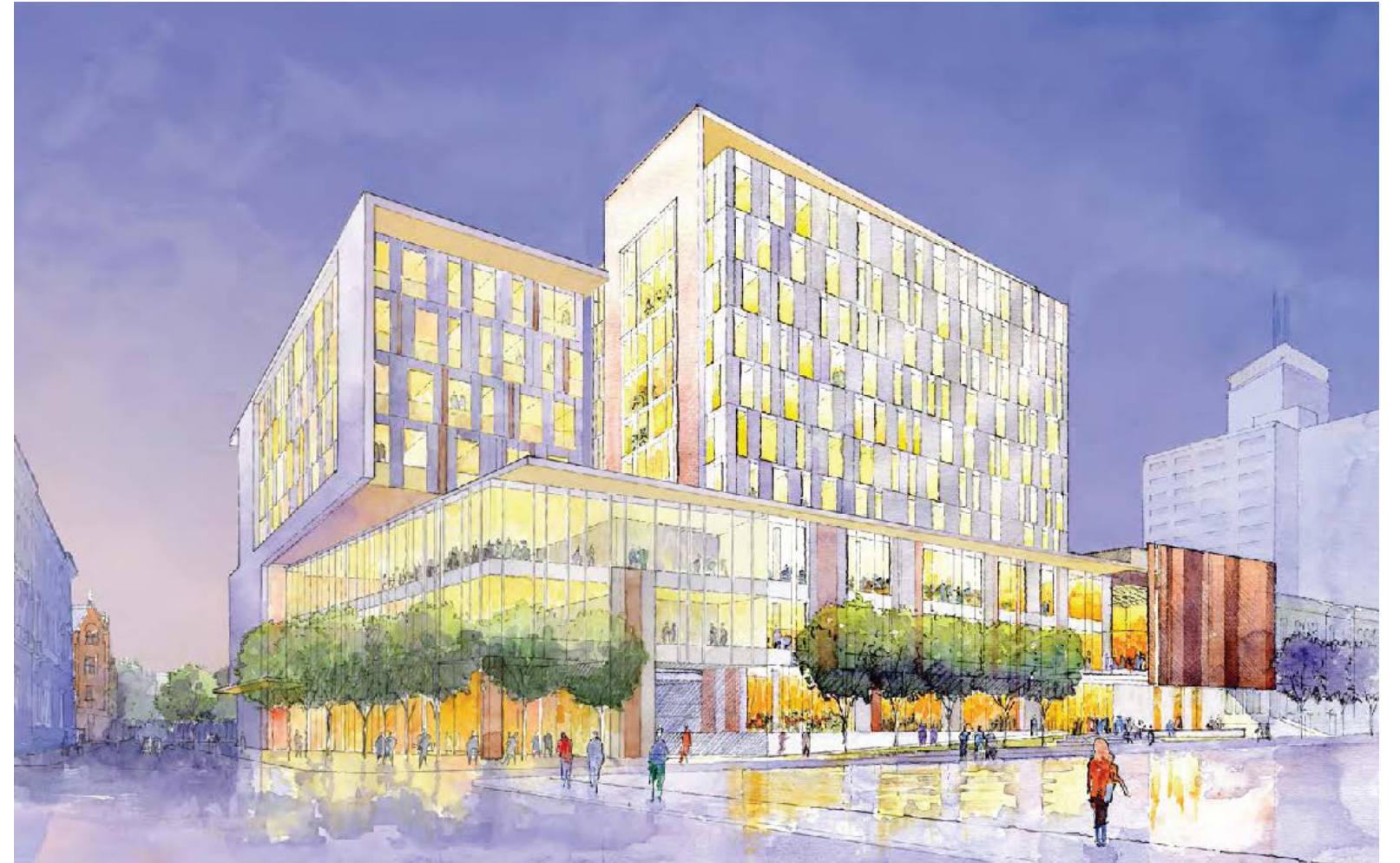
View of proposed NEC redevelopment, looking north from the intersection of Gainsborough and St Botolph Streets
