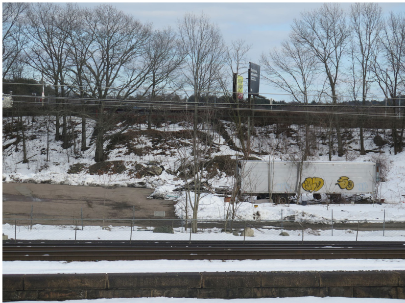
Existing Site From Across AMTRAK Main Line
