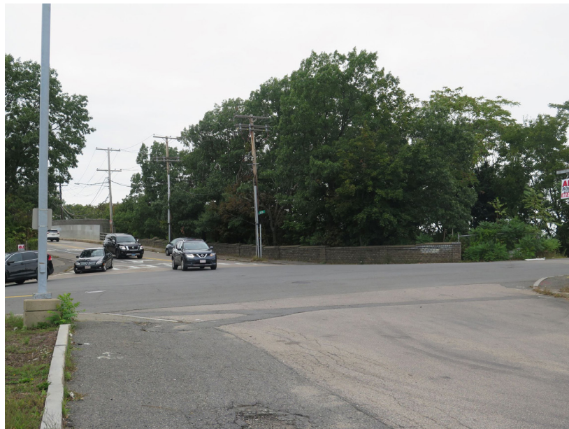
Milton Street Bridge and Hyde Park Avenue
