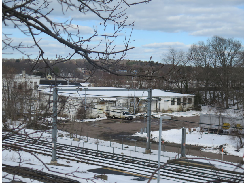
Existing Site Building From Across AMTRAK Main Line
