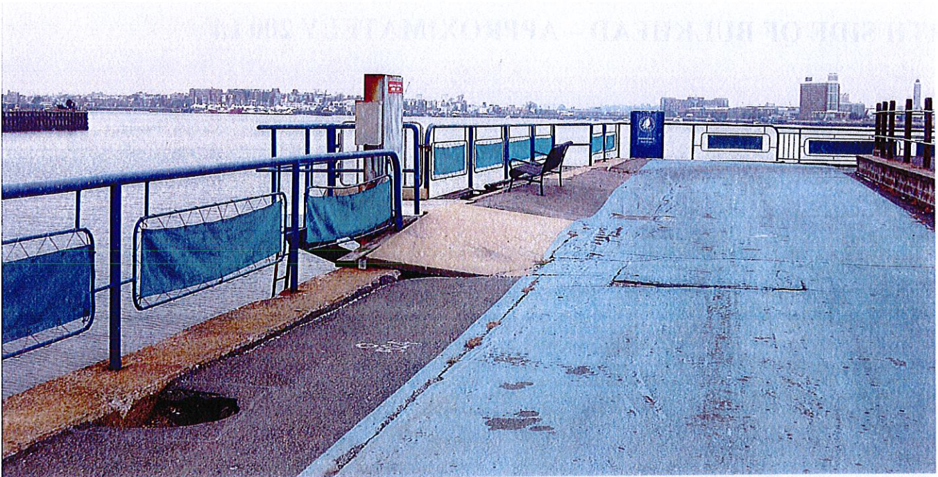
View of northwest corner of wharf 8's topside, looking north.
