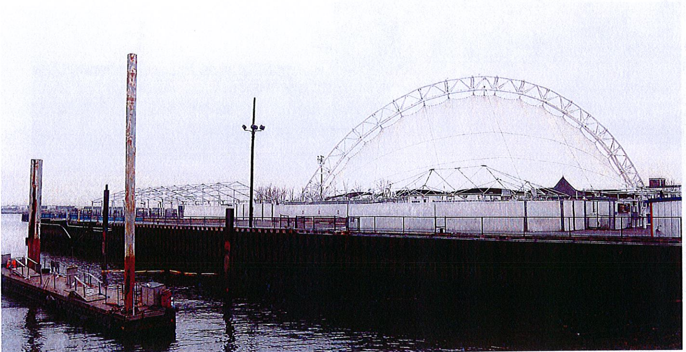
View of west side of Wharf 8 bulkhead
