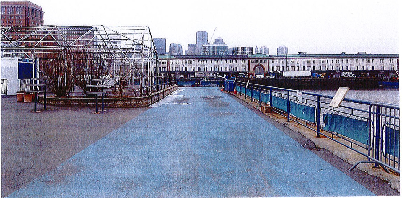
View of topside of north section of Wharf 8 bulkhead, looking west.
