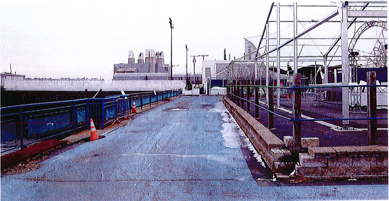
View of topside of north section of Wharf 8 bulkhead, looking east.
