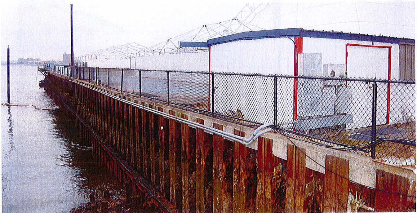
View of bulkhead and utilities, fencing and structures along west side.
