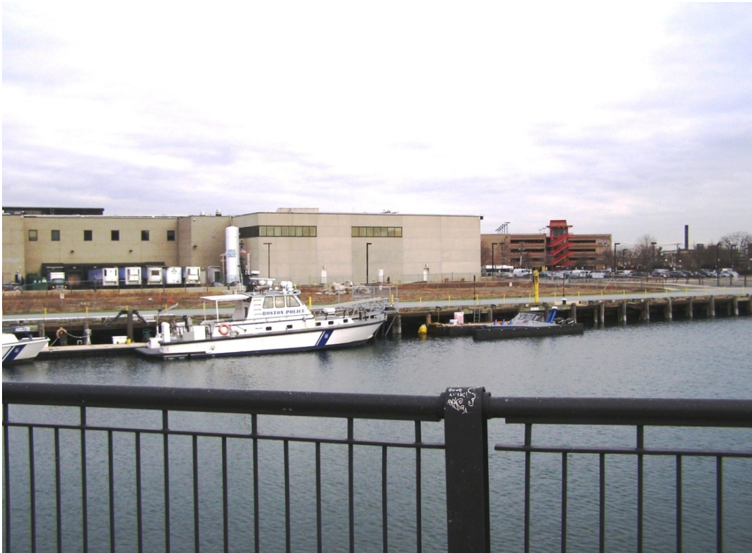
C-1, Berth 10, Northcoast Seafood Building from Summer Street Bridge
