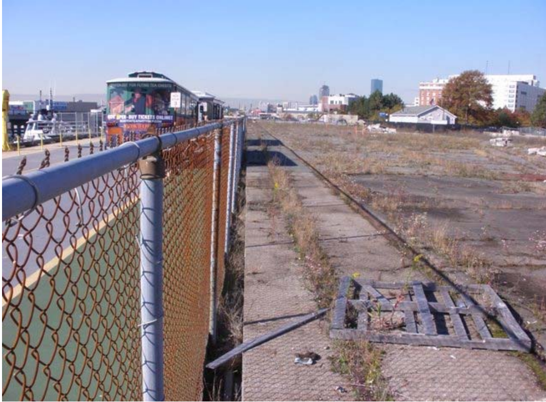
Berth 10/ Parcel C-1 (rear wharf)
