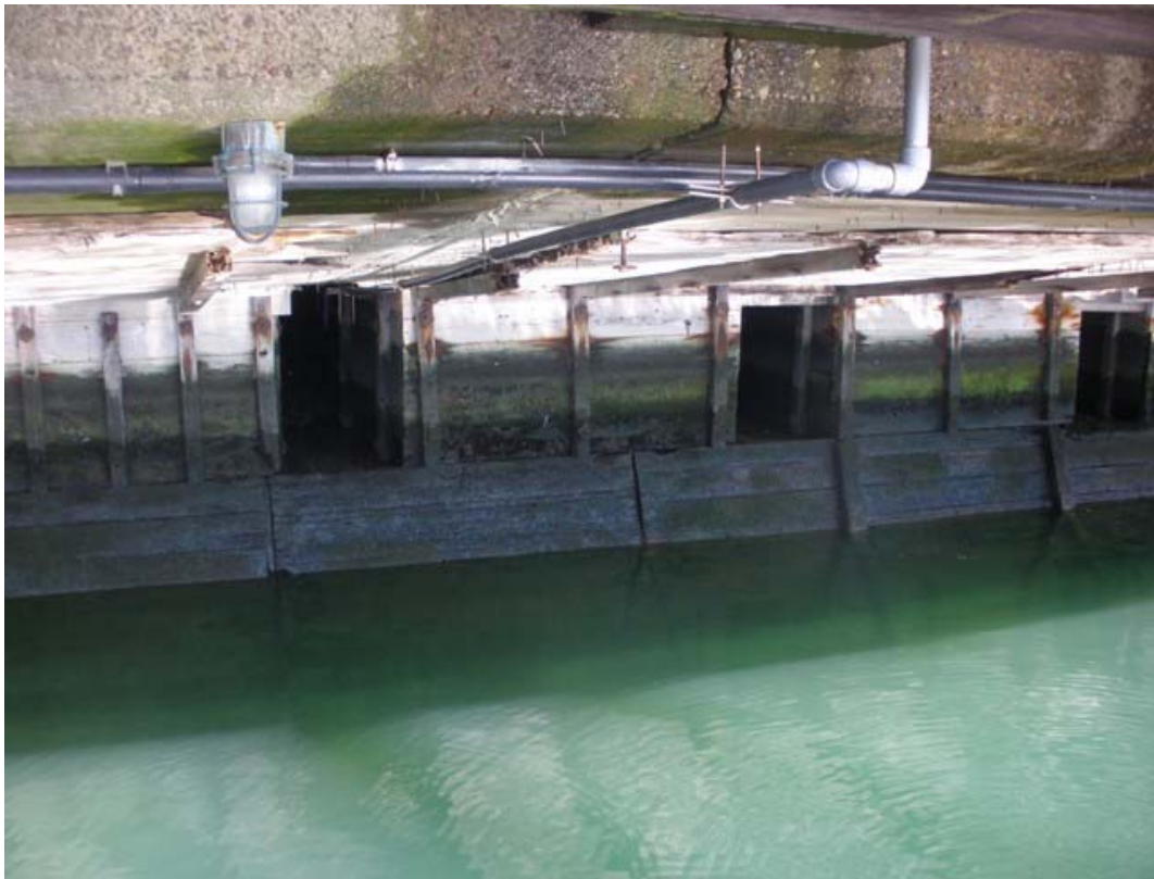
Drain openings beneath Berth 10 Access Road (front wharf)
