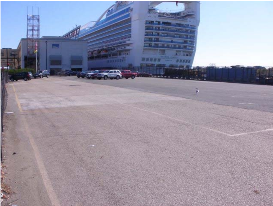
Parcel C-2 looking across southeast toward Massport Cruise Terminal with cruise ship at port
