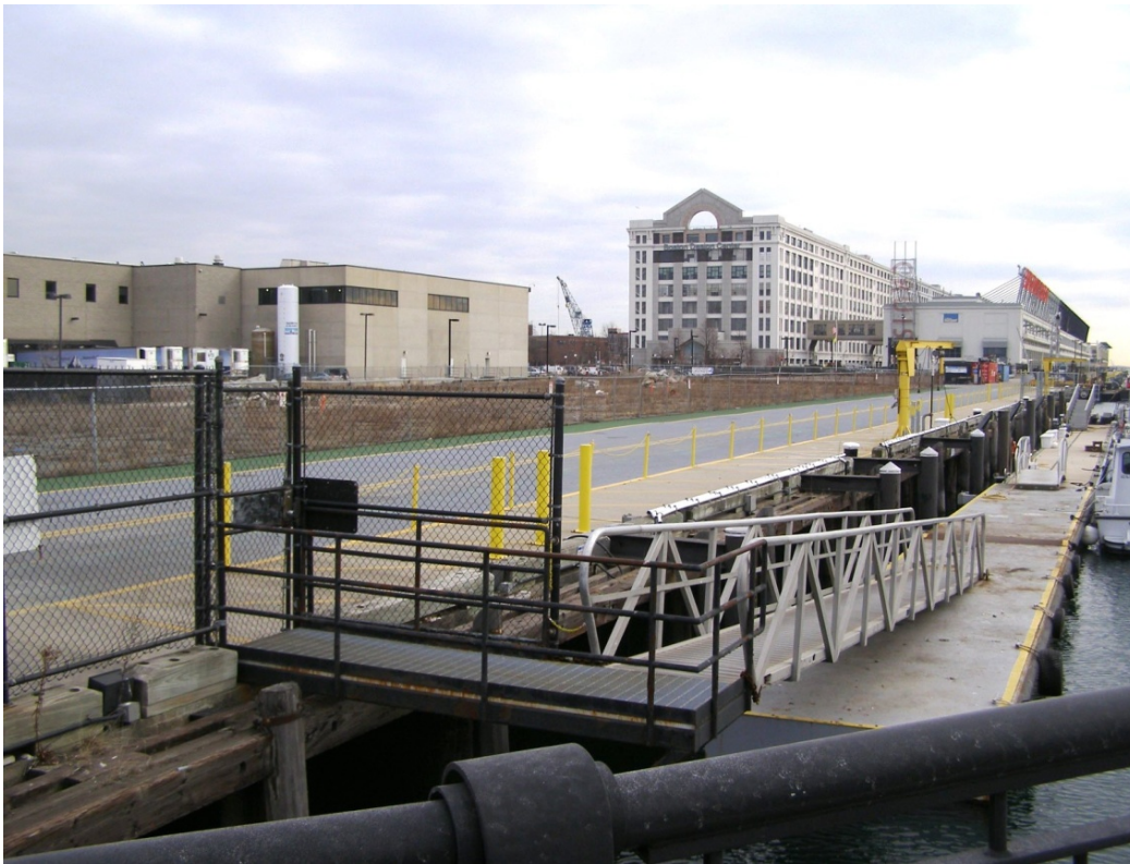
Berth 10/Reserve Channel wharf and floats
