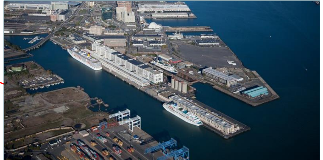
Raymond Flynn Industrial Park | South Boston Flood Mitigation Planning & Feasibility Study in-progress
