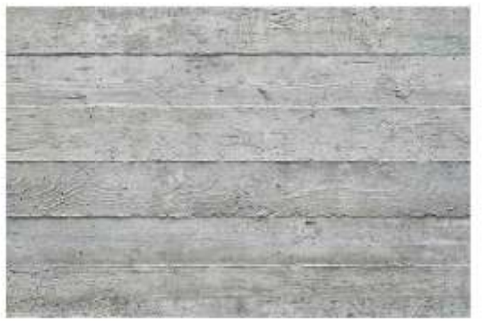
BOARD-FORMED CONCRETE FOUNDATION
