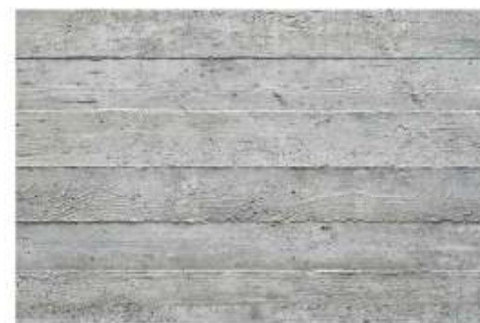
BOARD-FORMED CONCRETE FOUNDATION
