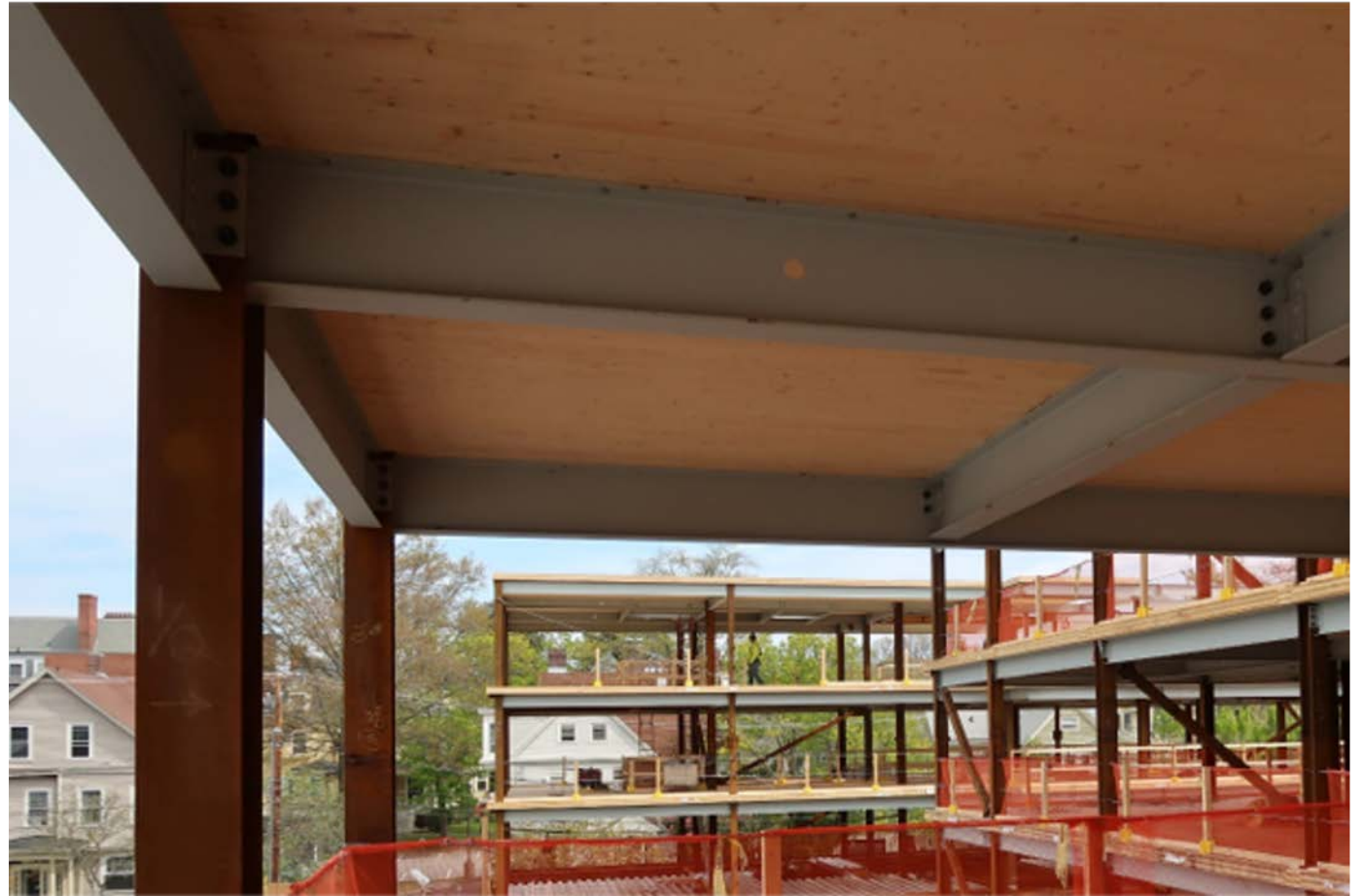
Mass Timber Hybrid – CLT deck panels and steel beams and columns
