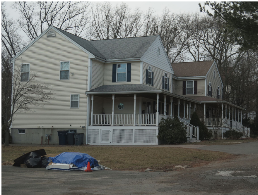
Adjacent Buildings at the End of Heron St
