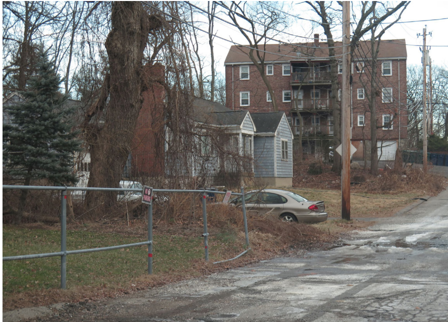
On-Site Building at 11 Heron St and Adjacent 4907 Washington St
