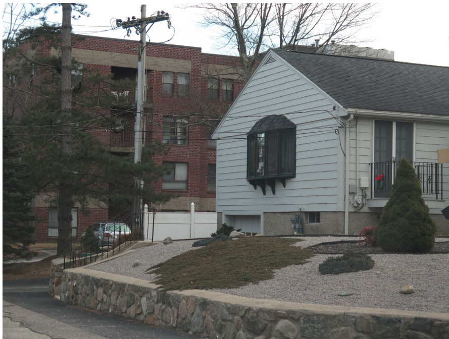
On-Site Building at 26 Heron St and Adjacent Stony Brook Condominiums
