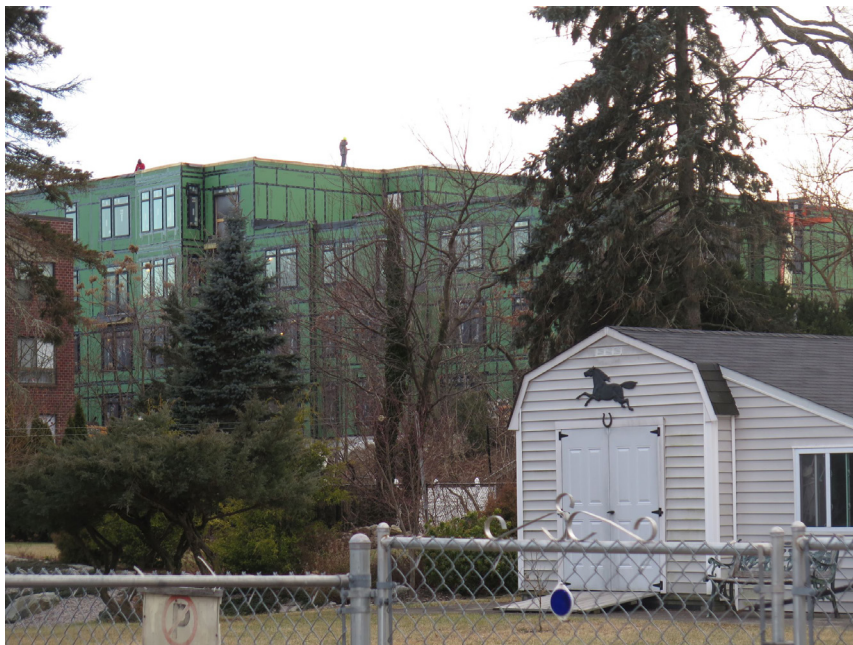
Adjacent New Development (Under Construction) on Willet St
