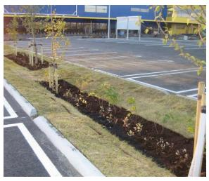
Natural infiltation of stormwater is facilitated by bioswales, such as these at a retail store parking lot.
