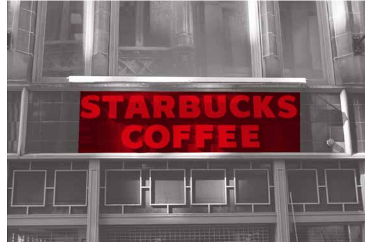
Flat sign with projecting letters on building material.
