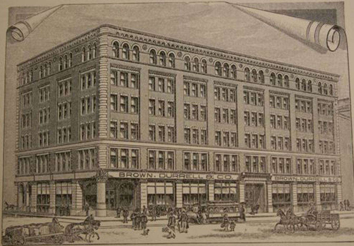
BUILDING CORNER OF ESSEX AND KINGSTON STREETS.
