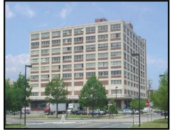
12 Channel St Building
