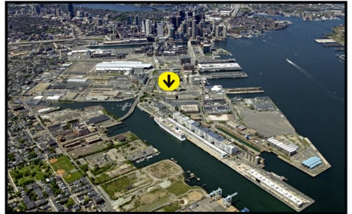
Boston Marine Industrial Park
