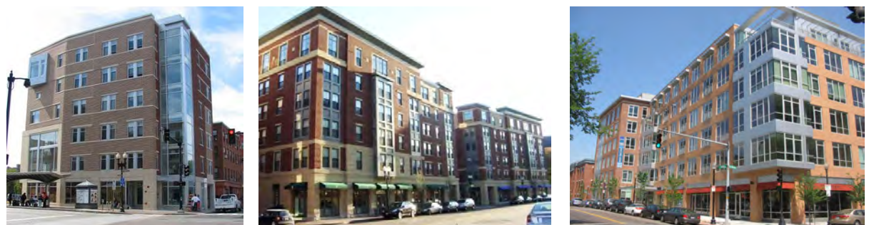
The stepbacks, window and corner details, and cornice lines help to articulate these buildings.
