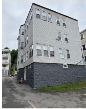
EXISTING REAR / EAST VIEW
