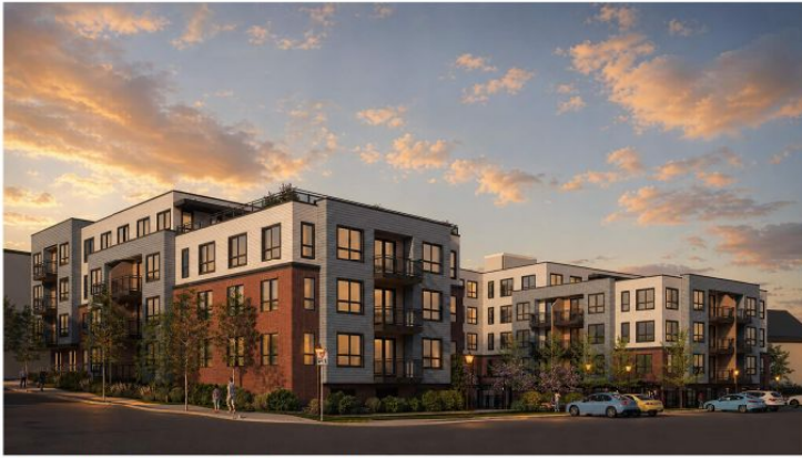
VIEW APPROACHING FROM WASHINGTON ST.
