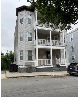
EXISTING FRONT VIEW, GOODALE ROAD
