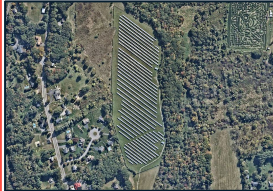
2.4 MW Ground-Mounted Solar - Sterling, MA
