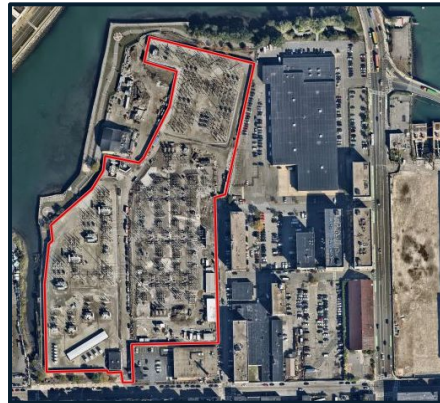
K Street Substation in South Boston, MA
