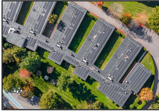
537 kW Roof-Mounted Solar - Jamaica Plain, MA
