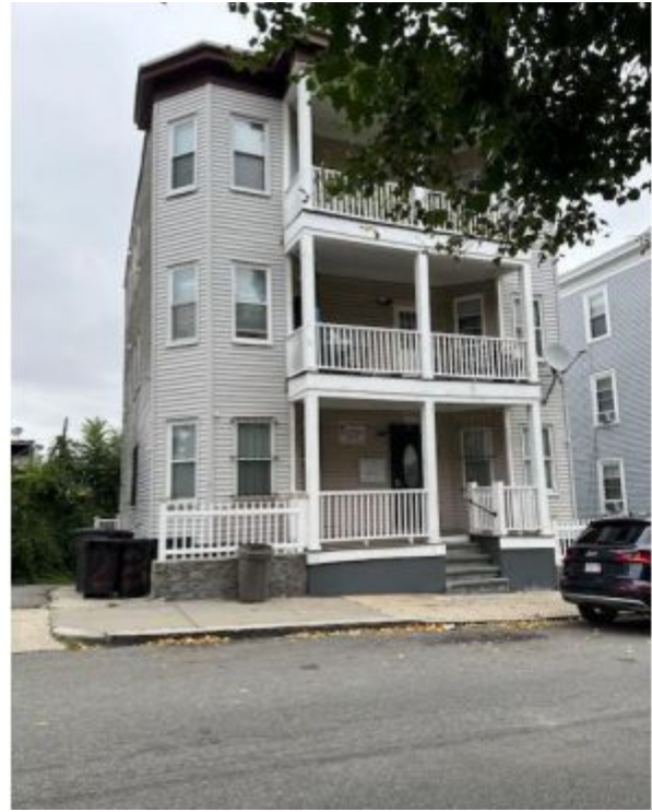
EXISTING FRONT VIEW, GOODALE ROAD
