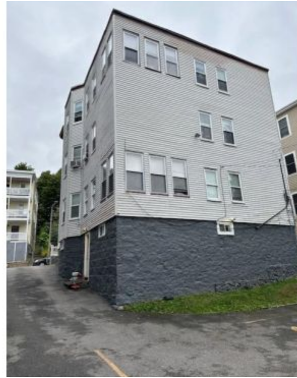
EXISTING REAR / EAST VIEW
