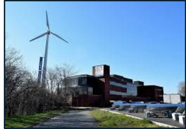
100 kW Wind Turbine - Dorchester
