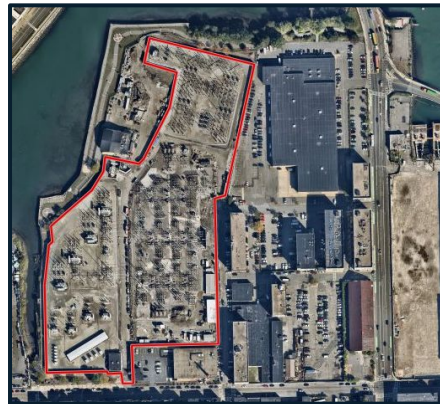
K Street Substation in South Boston, MA
