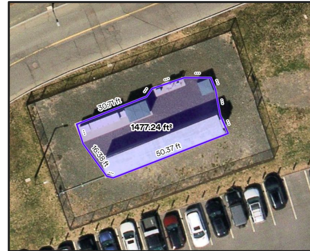
UMass Amherst Central Heating Plant - Amherst, MA
