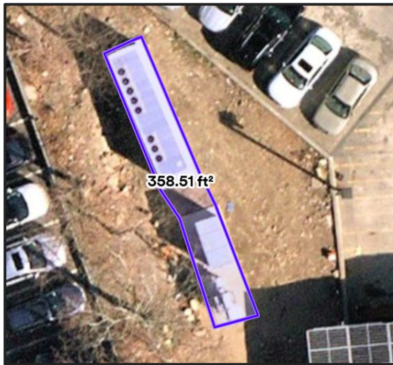
Mamaroneck Avenue School BESS - No fenced perimeter at all
