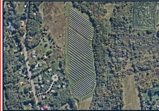
2.4 MW Ground-Mounted Solar - Sterling, MA
