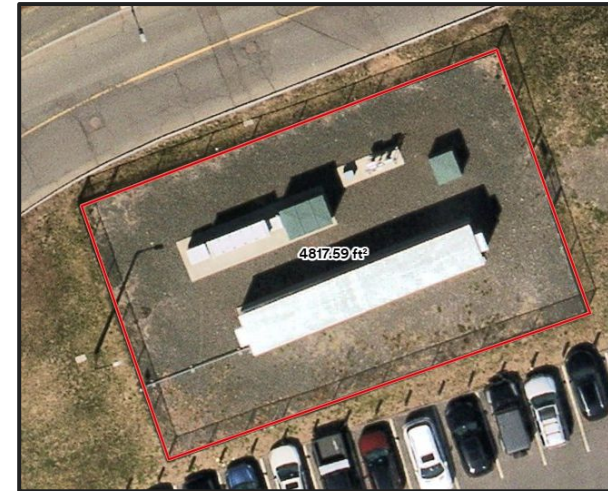
UMass Amherst Central Heating Plant - Amherst, MA
