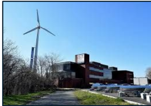
100 kW Wind Turbine - Dorchester
