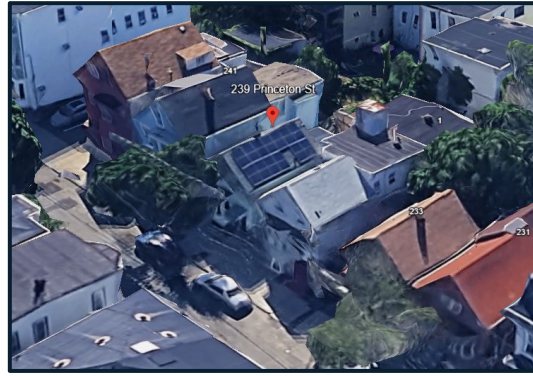
3.8 kW Roof-Mounted Solar - East Boston, MA
