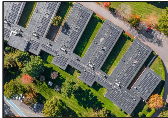
537 kW Roof-Mounted Solar - Jamaica Plain, MA
