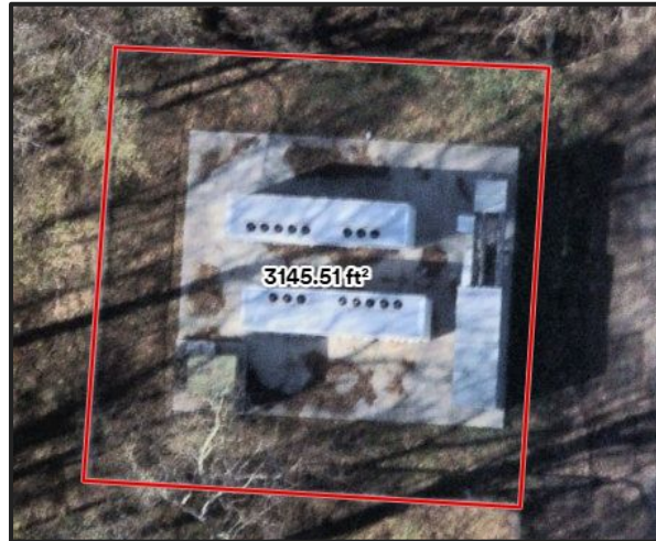
Gedney Way Recycling Facility - White Plains, NY
