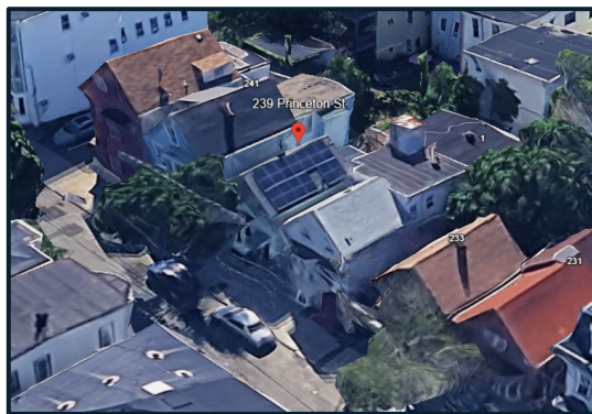
3.8 kW Roof-Mounted Solar - East Boston, MA
