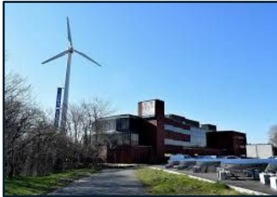
100 kW Wind Turbine - Dorchester
