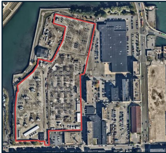
K Street Substation in South Boston, MA
