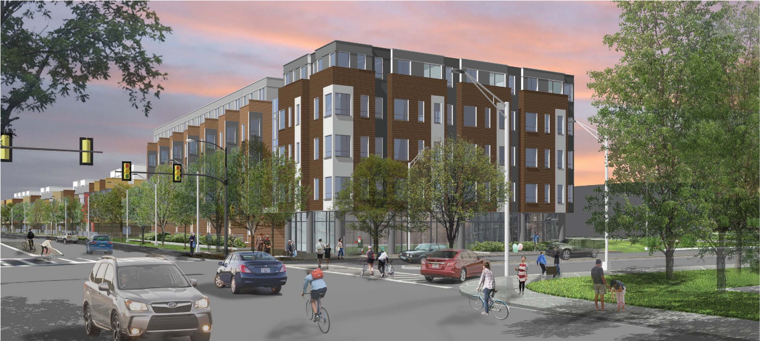
Southwest View of the Five Story Apartment Building (Near Ukraine Way and Hyde Park Avenue Intersection)
