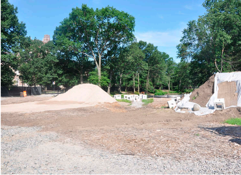
Figure 3. Emerald Necklace - West Fens, under construction
