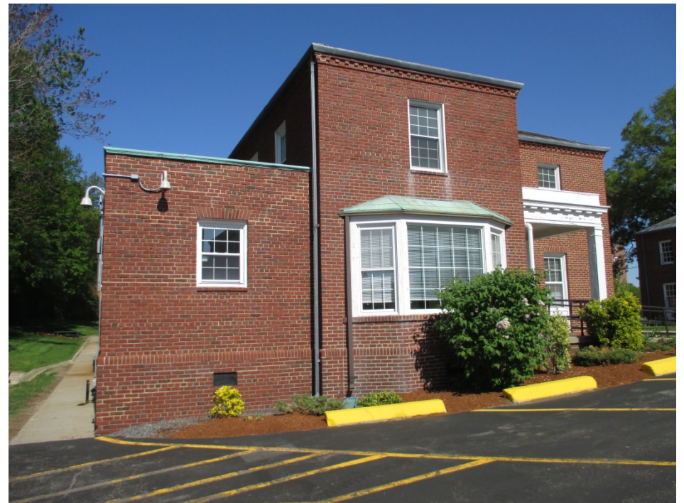
15. Building 4, view west of east elevation
