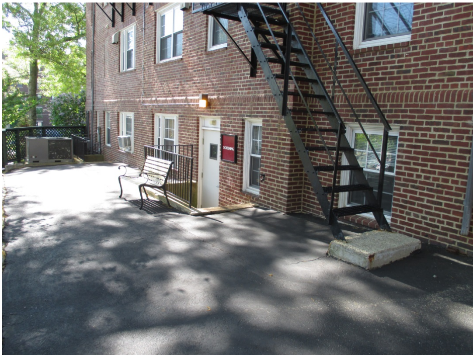
32. Building 6, view southeast of north elevation
