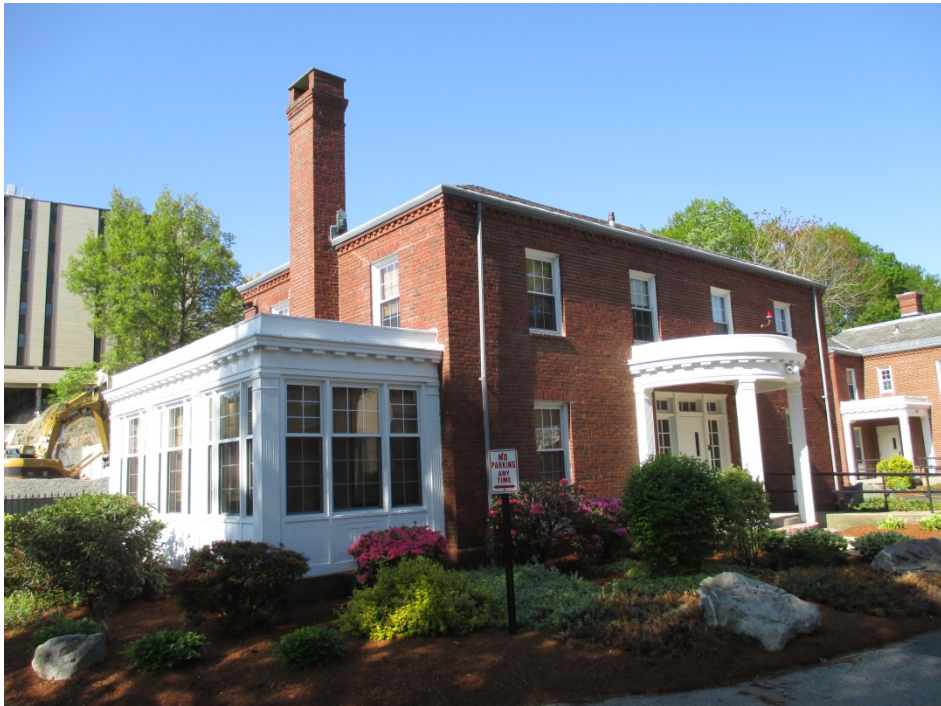
3. Building 3, view southwest of north and east elevations, building to remain
