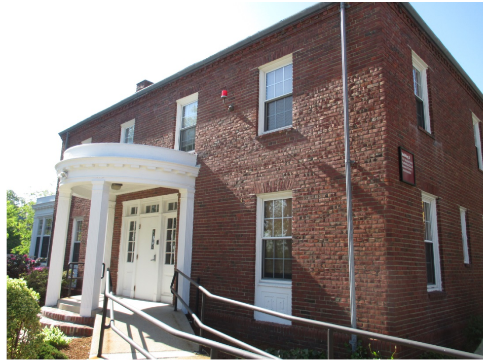
2. Building 3, view southeast of north and west elevations, building to remain
