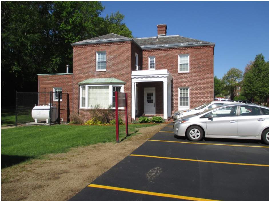
24. Building 5, view west of east elevation
