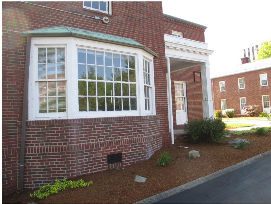
37. Building 7, view southeast of west elevation
