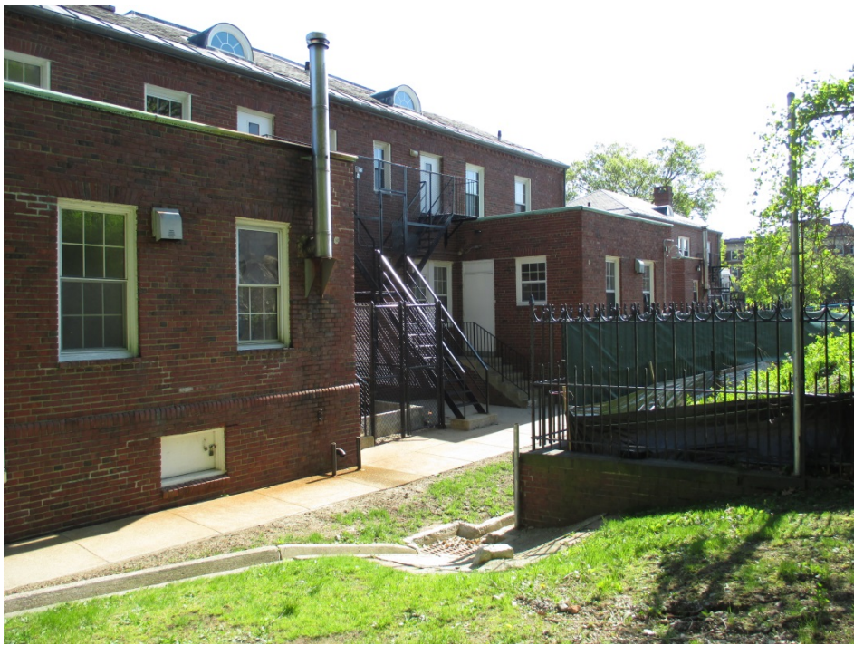
12. Building 4, view northeast of south elevation
