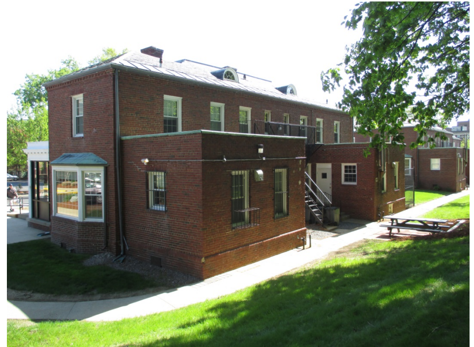
21. Building 5, view northeast of west and south elevations
