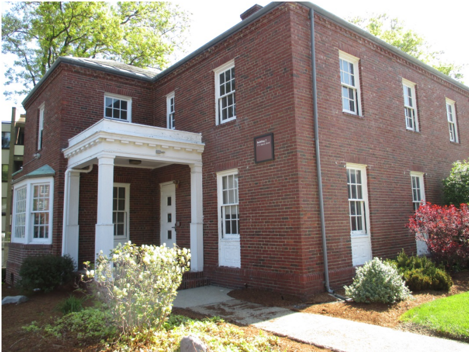
35. Building 7, view northeast of west and south elevation
