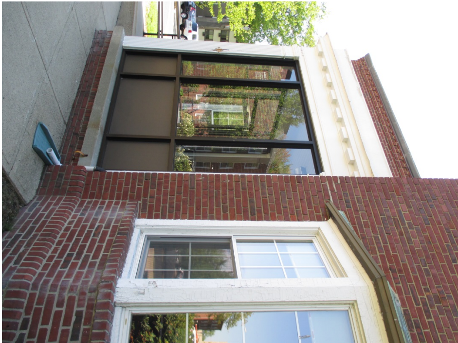
20. Building 5, view northeast of infill at entrance off west elevation
