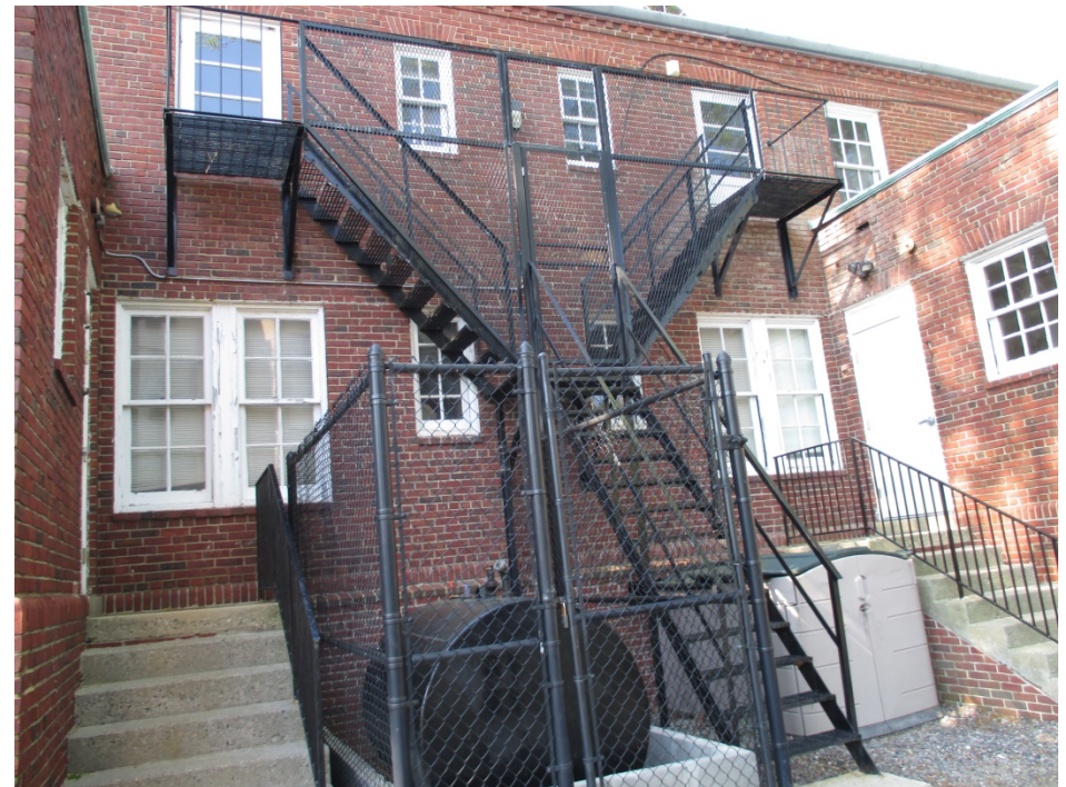
40. Building 7, view south of north elevation
