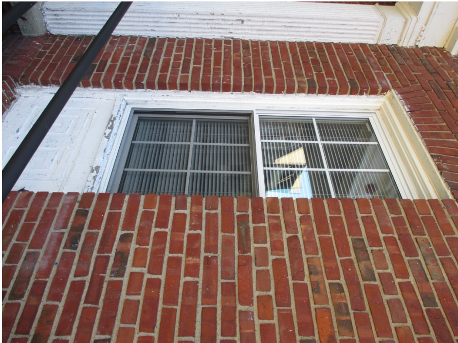
28. Building 6, view northeast of west elevation window
