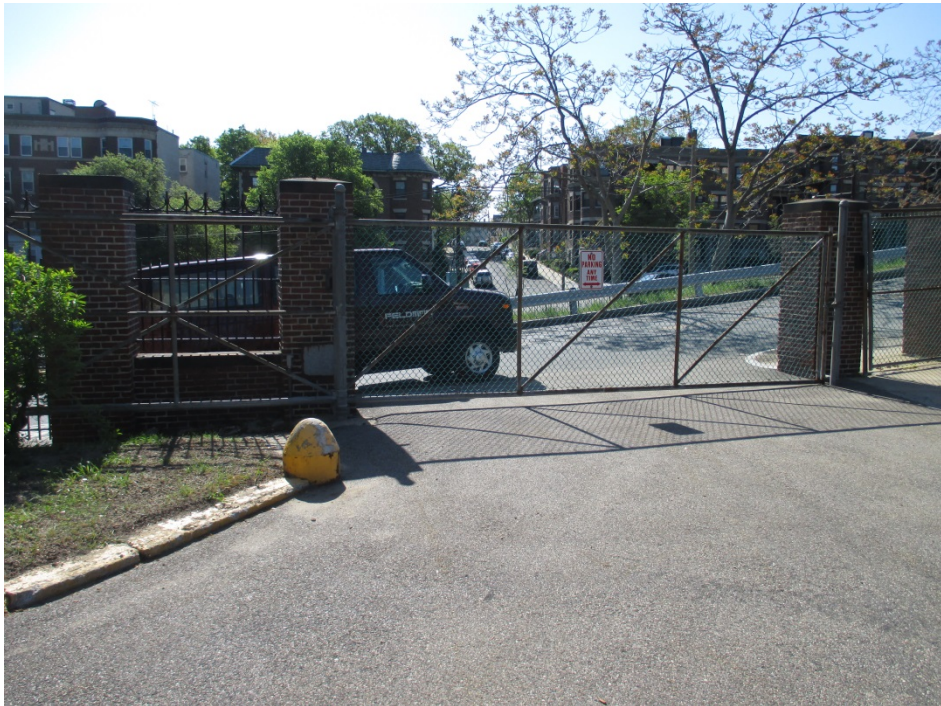
43. Site, view east of entrance gate
