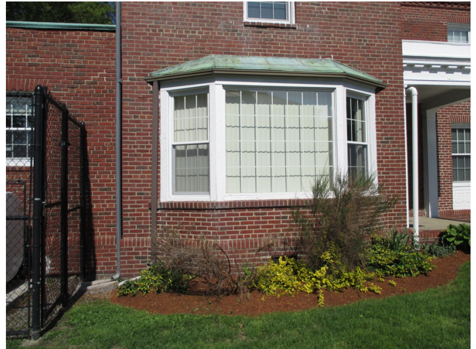
25. Building 5, view west of east elevation, window
