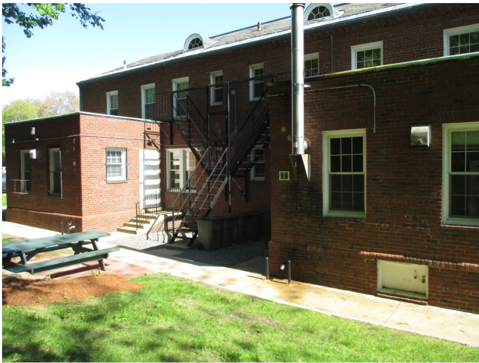
22. Building 5, view northwest of south elevation
