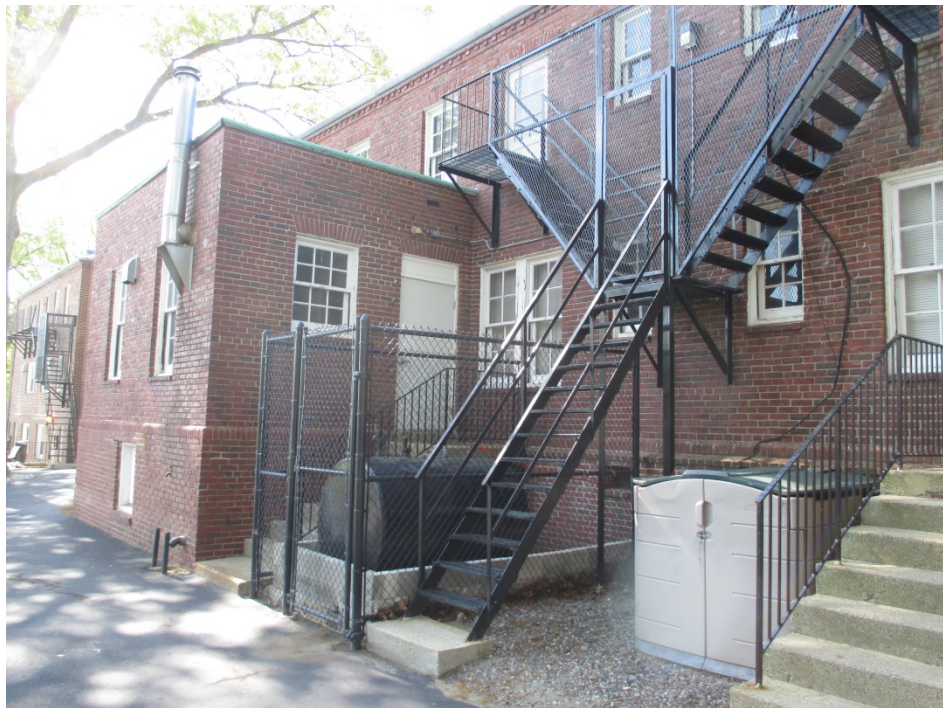
39. Building 7, view southeast of north elevation
