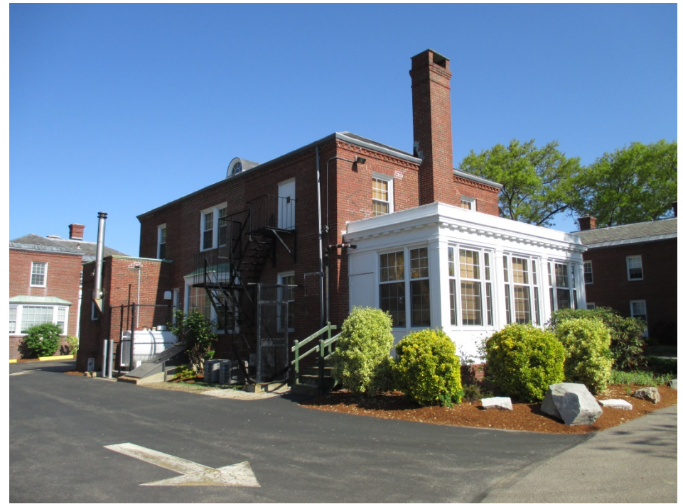
6. Building 3, view northwest of south and east elevations, building to remain
