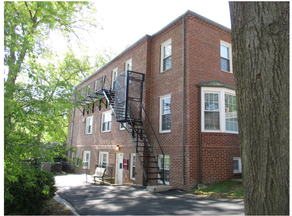
31. Building 6, view southeast of north elevation
