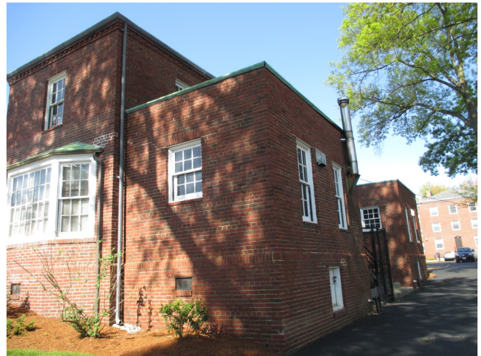
38. Building 7, view southeast of west and north elevations
