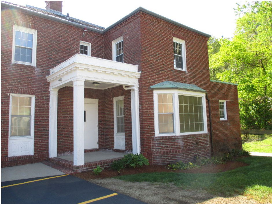
10. Building 4, view southeast of west elevation
