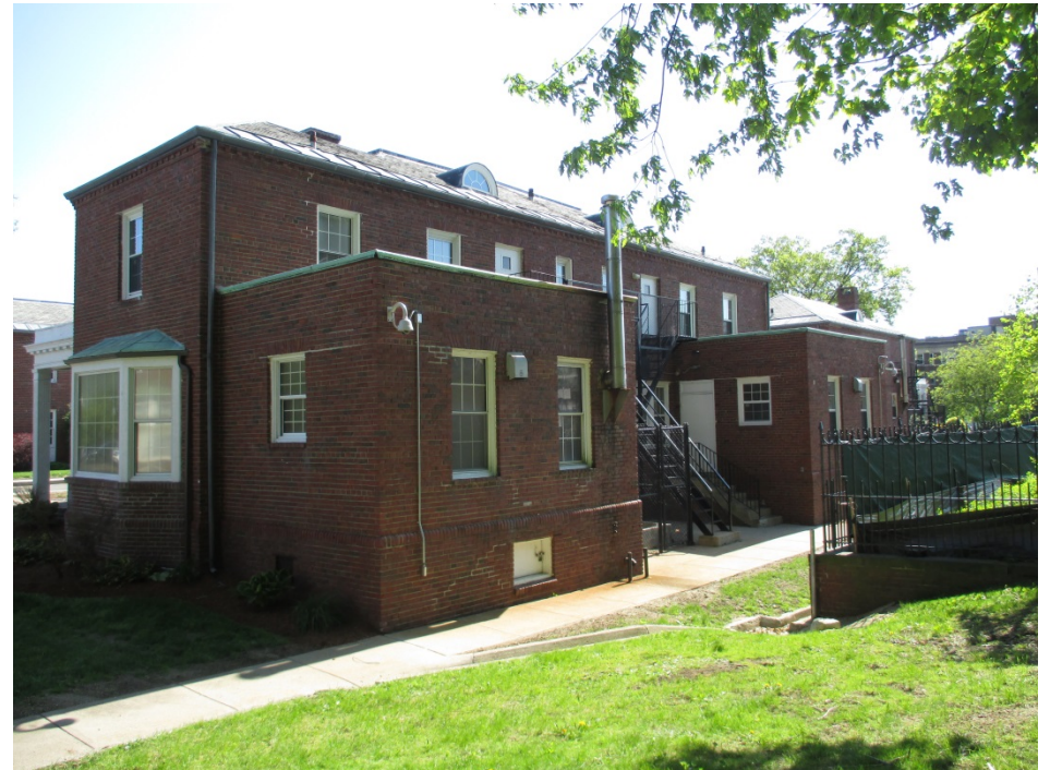
11. Building 4, view northeast of west and south elevations
