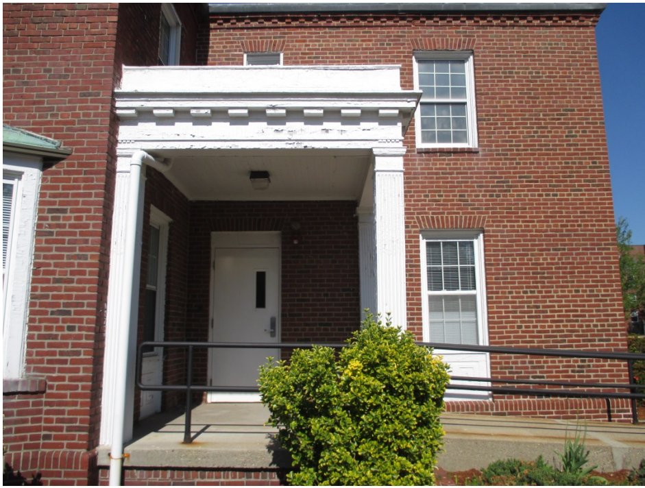
16. Building 4, view south of north elevation entrance
