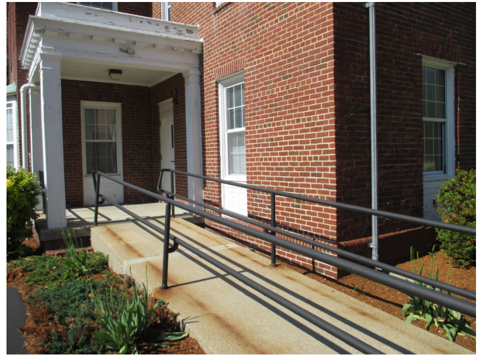
17. Building 4, view west of east elevation at entrance
