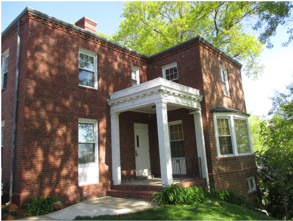
30. Building 6, view northwest of east elevation
