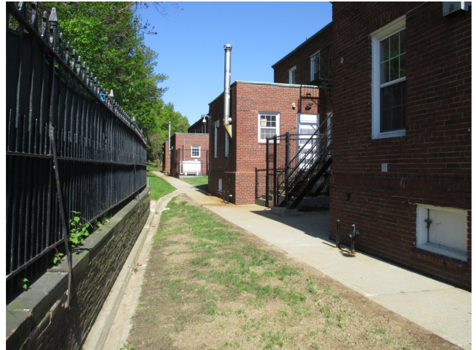
44. Site, view west of south walkway from Building 3
