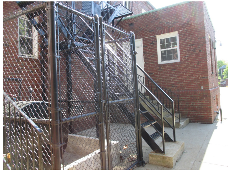
13. Building 4, view northeast of south elevation, fire escape
