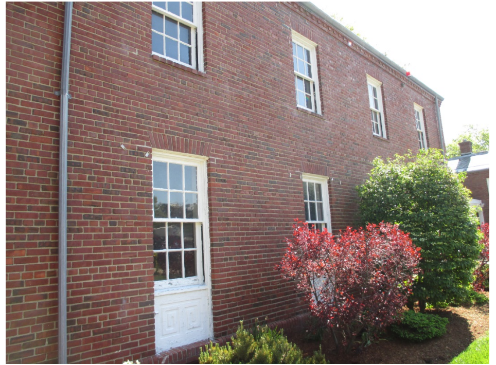
34. Building 7, view northeast of south elevation
