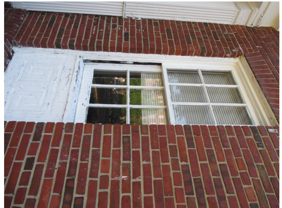
36. Building 7, view northeast of east elevation window
