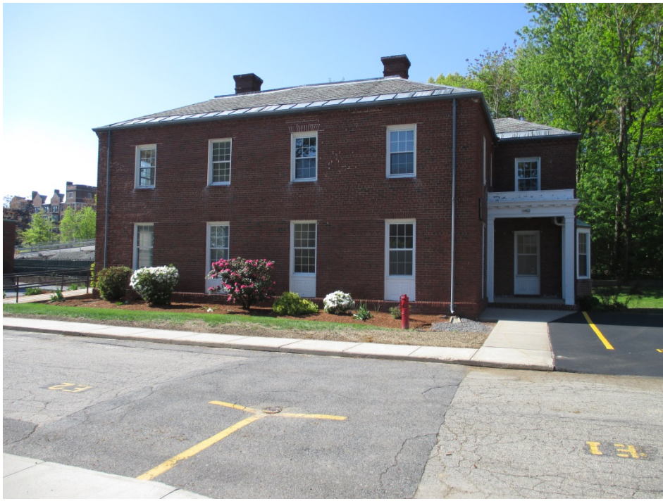
8. Building 4, view south of north elevation
