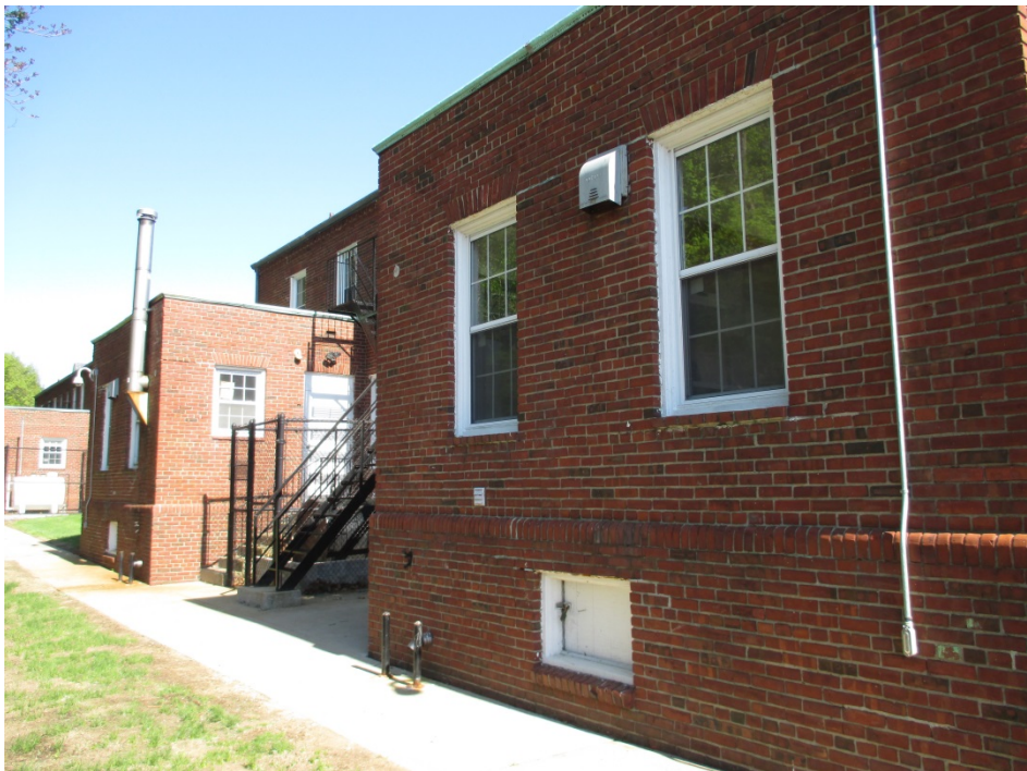
14. Building 4, view northwest of south elevation
