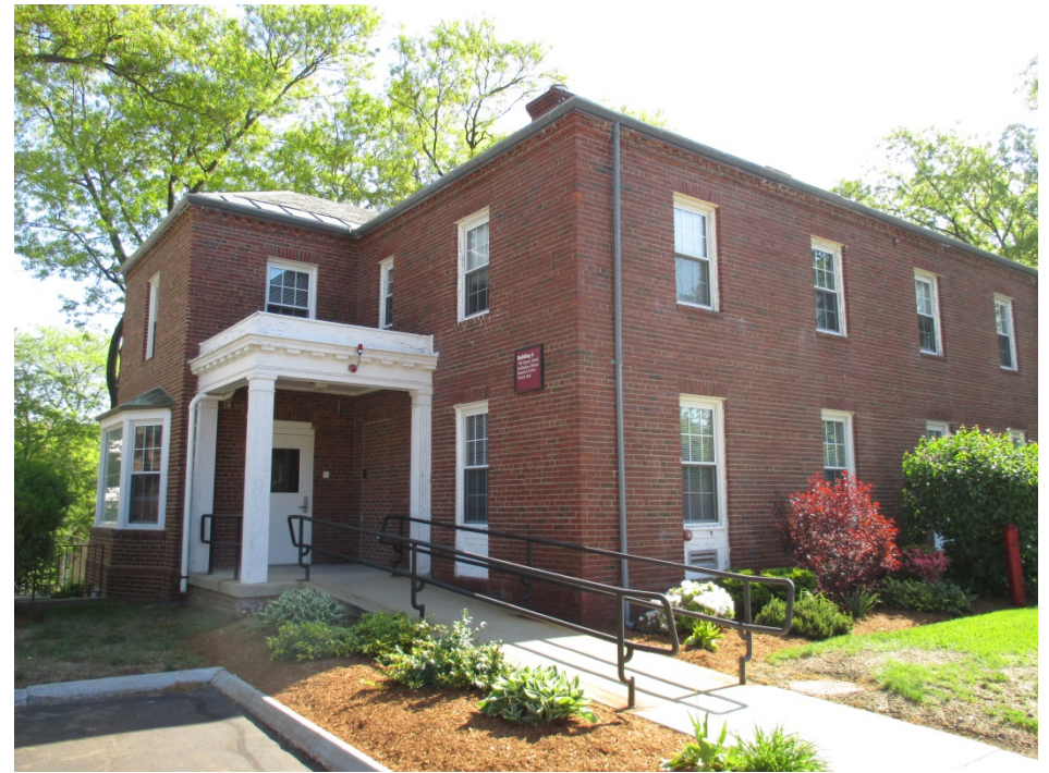
27. Building 6, view northeast of west and south elevations
