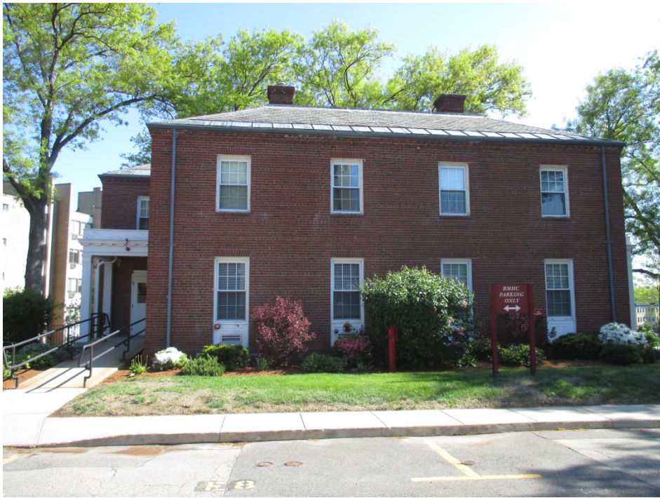
26. Building 6, view north of south elevation
