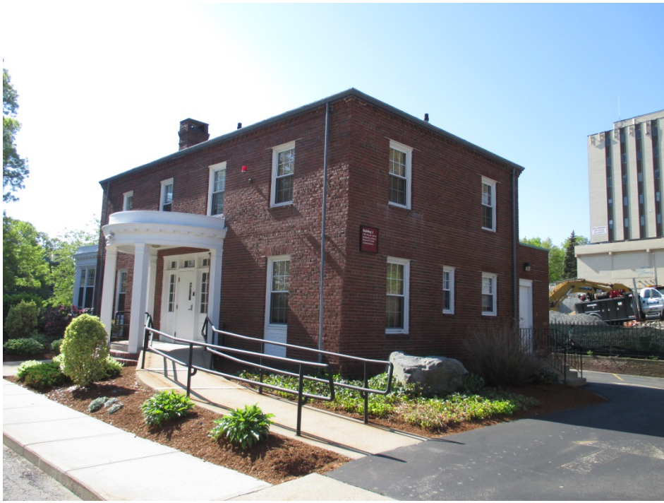
1. Building 3, view southeast of north and west elevations, building to remain
