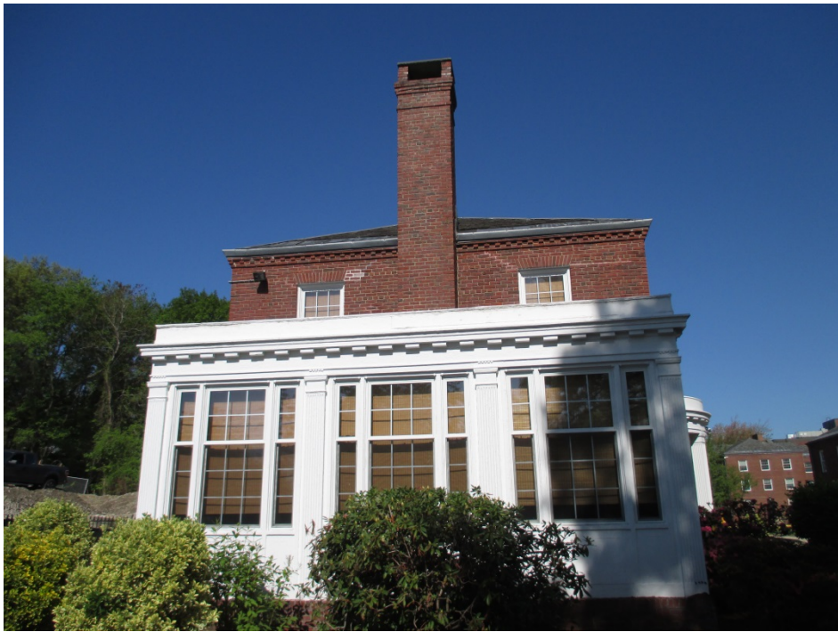
5. Building 3, view west of east elevation, building to remain
